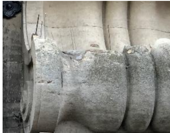
Spalling stonework
