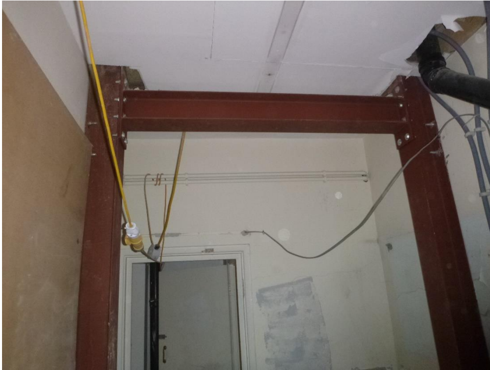
Steel frame inserted internally adjacent to flank wall
