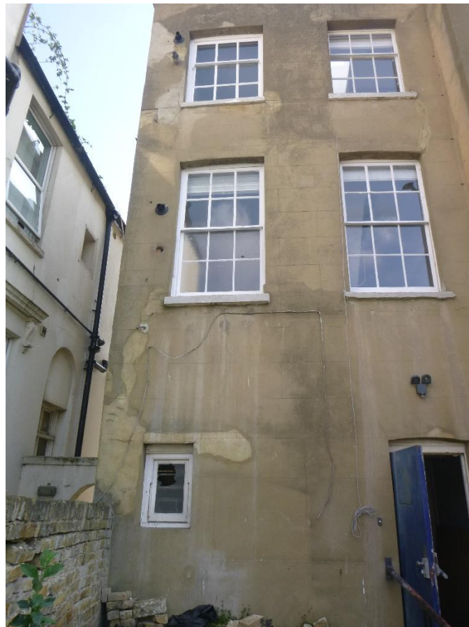
Rear elevation adjacent to flank wall
