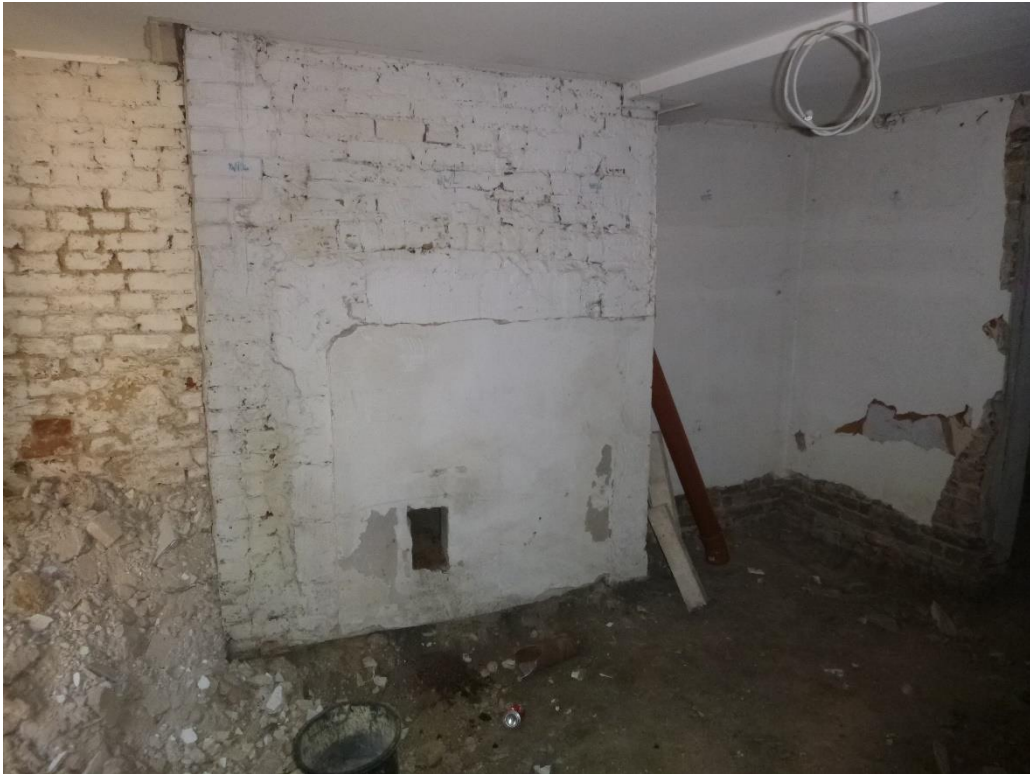
Excavations in basement showing shallow footings to chimney on party wall
