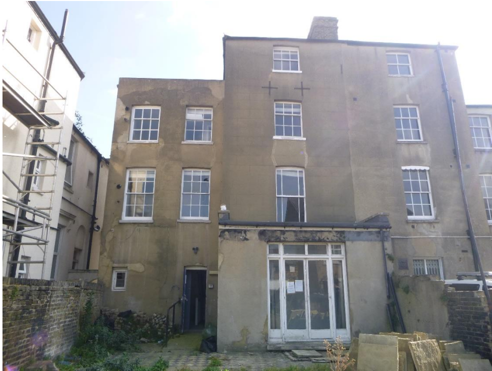
Rear elevation (Historic ties at 3 rd Floor level)
