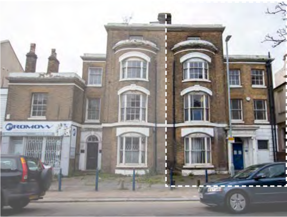
Left - adjoining building 196/7 Right - application building 195 Parrock Street Photo from Historic England by C Watson 8/3/20
