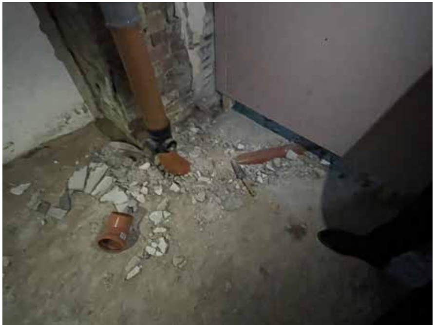
View C - Basement finished floor depicting new waste run and SVP
