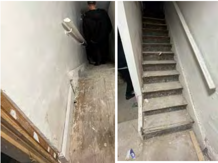
No. 195 GF to LGF Noteworthy: floorboards in tack. Evidence of new skirting and architrave being formed to previously utilised GF WC (proposed to provide inner access to passageway in JCA scheme)
