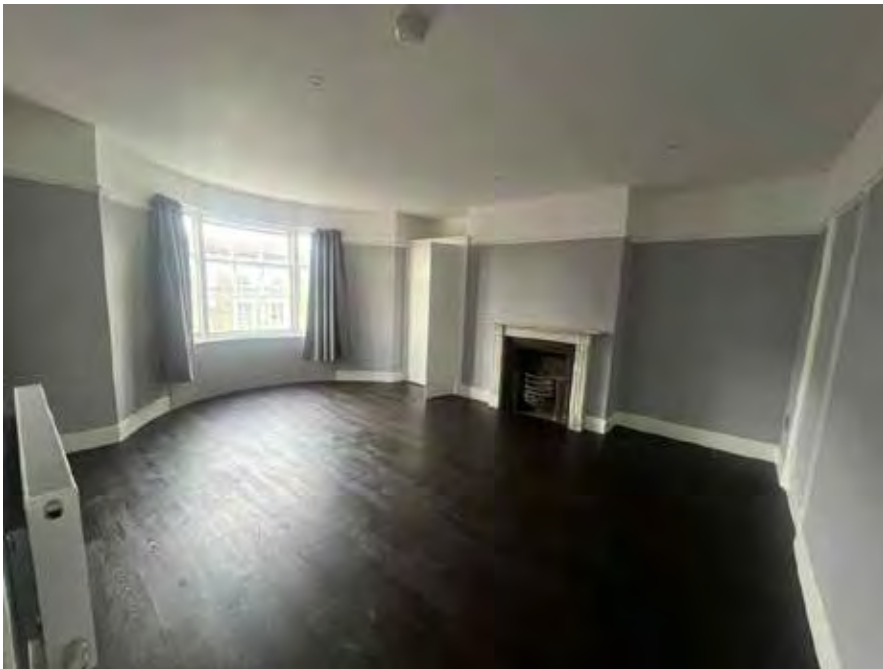
View D - No. 195 third floor interior - front living room looking south Noteworthy fireplace, mantel, window, sill, skirting and architrave intact Drawing not to scale - for publication purposes only
