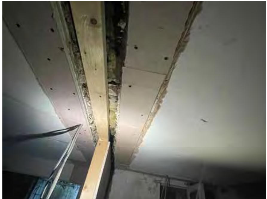
View D - No. 195 Basement partitions being installed prior to aborted work. Evidence of construction methods, timber stud, fire rated gypsum plasterboard,
