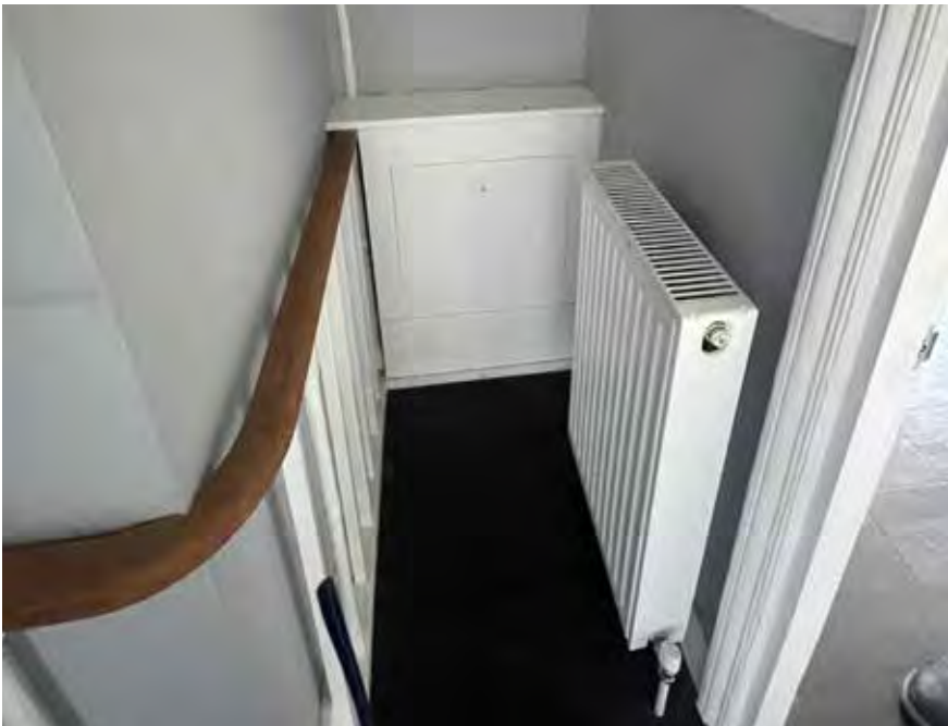
No. 195 2f landing - note balustrade and spindles remain in situ behind partition Noteworthy: solid partition infill (noted as glazed in Section 73 drawings)
