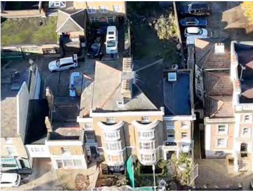
Looking west - No. 195 & 6 forming a pair with matching hipped slate roofs over wings, evidence of No. 195 later flat roof extension to the north
