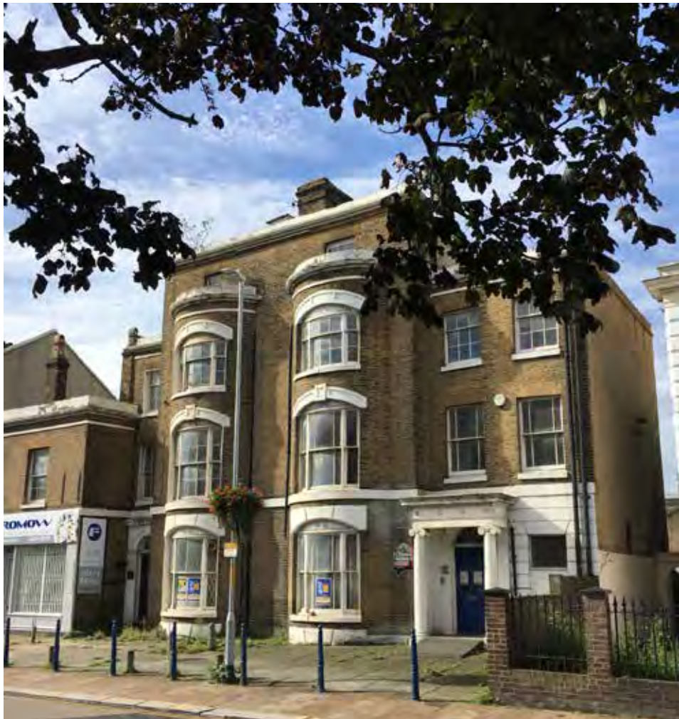
195 (centre) & 196/197 (left) front elevation 194 cast iron painted barriers to right Painted Local Authority bollards to front Photo from Historic England by Charles Watson 8/3/20
