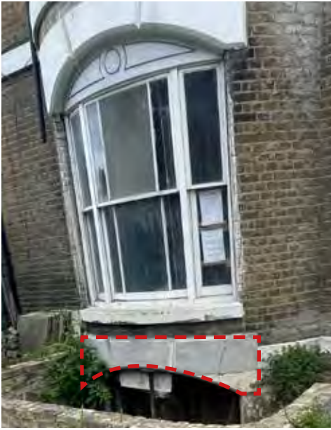
Front ground floor bay and window with stone lintel to basement lightwell aperture below
