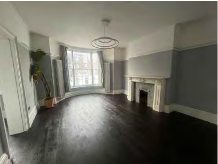
View D - Front living room looking east toward bow window Noteworthy - window, architrave, picture rail and skirting in tack. Drawing not to scale - for publication purposes only
