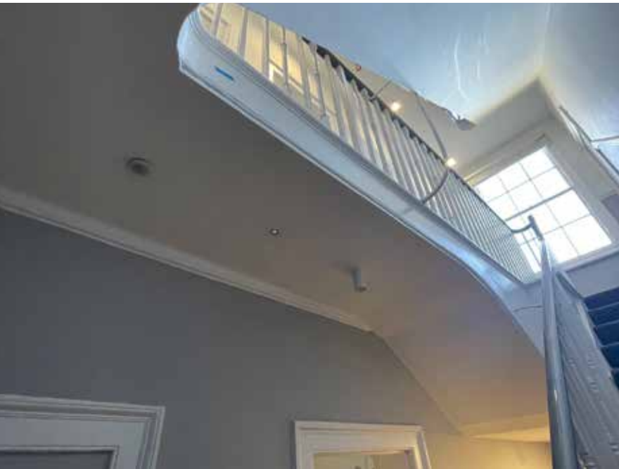
No. 195 GF to 1F Noteworthy: spindles, timber stringer and banister in tact. Historic architraves and coving in tact. Evidence of smoke alarms and lighting installed.
