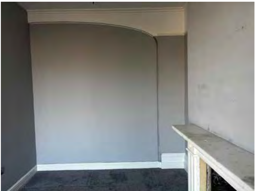
View B - Front living room interior looking west toward arch Noteworthy - arch in tack. Panel infill provides shadow gap
