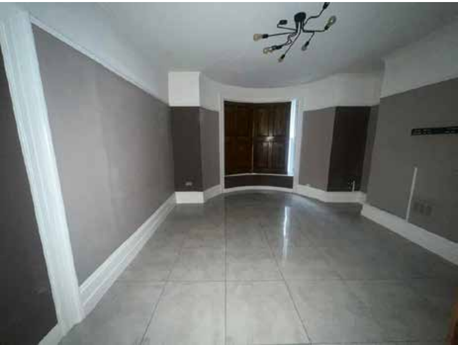
View A - No. 195 ground floor interior front living room looking east toward front bow window.. Note ceramic tiled floor. Evidence of architrave, skirting, cornice and dado intact.
