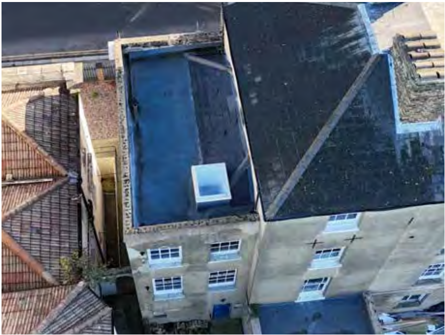
Looking east - No. 195 flat roof depicting roof light through historic pitched hipped slate roof, EPDM (or similar) surface treatment.
