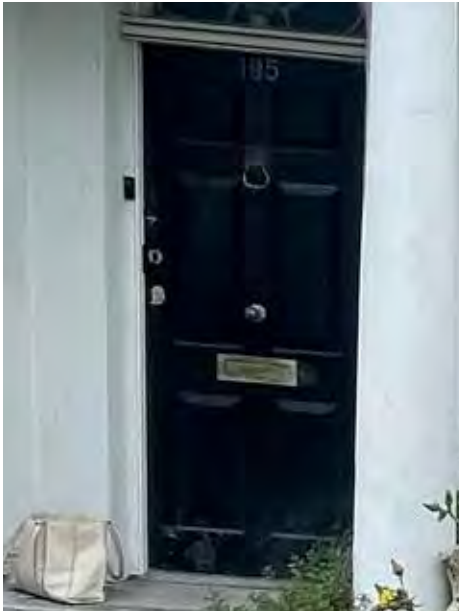
Existing main external entrance door to remain in situ
