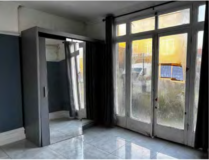
View D - No. 195 ground floor interior - rear bedroom looking west toward French doors French doors and side and top lights appear as existing not replaced
