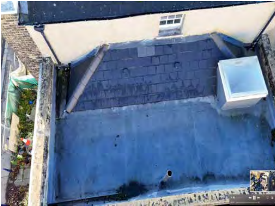
Looking south - No. 195 flat roof depicting SVP (assumed in same location since 1970's office wc's to second floor) Chimney removed. Roof vents assumed to be servicing
