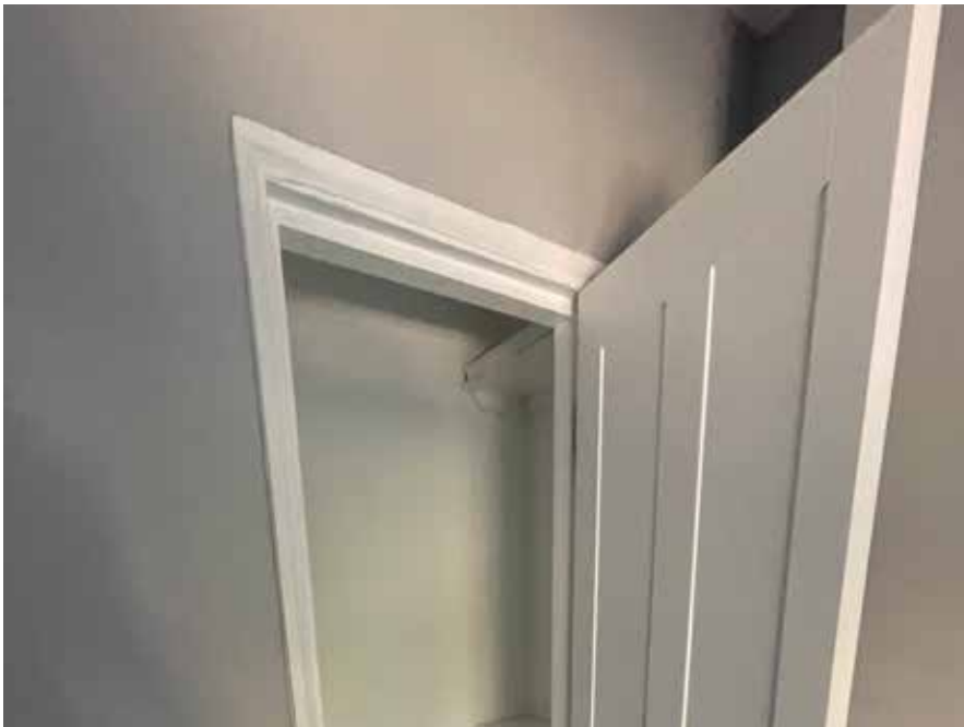
View B - No. 195 2F under stair cupboard
