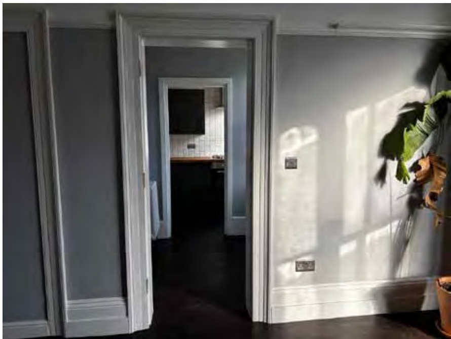
No. 195 second floor interior lobby - mid unit looking east. Noteworthy: architrave and skirting intact
