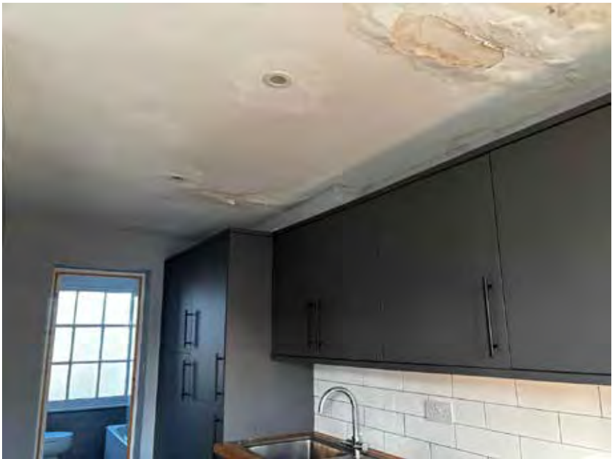
View A - No. 195 third floor kitchen to bathroom
