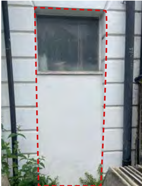
North wing extension later window (previous bank night deposit box aperture) To be replaced with side passage door
