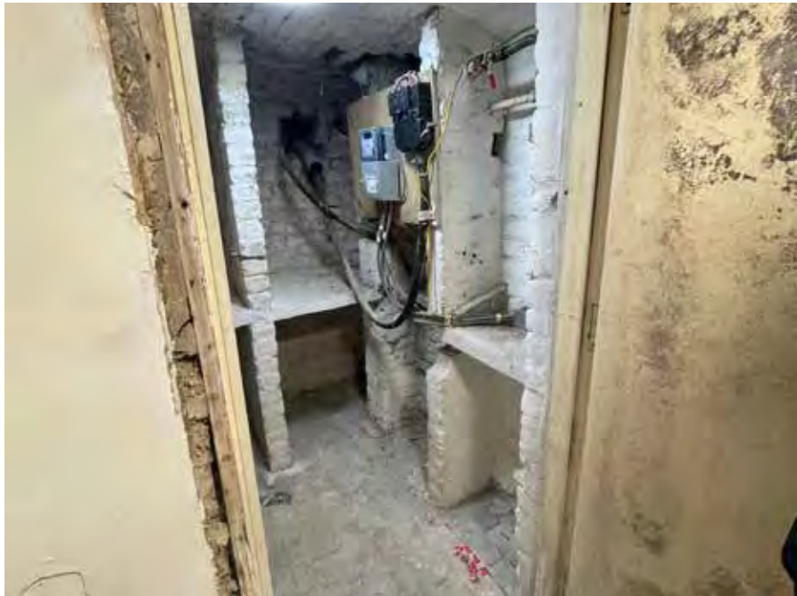
View B - No. 195 existing basement services cup. Noteworthy brick barrel ceiling, brick floor and divisions intact
