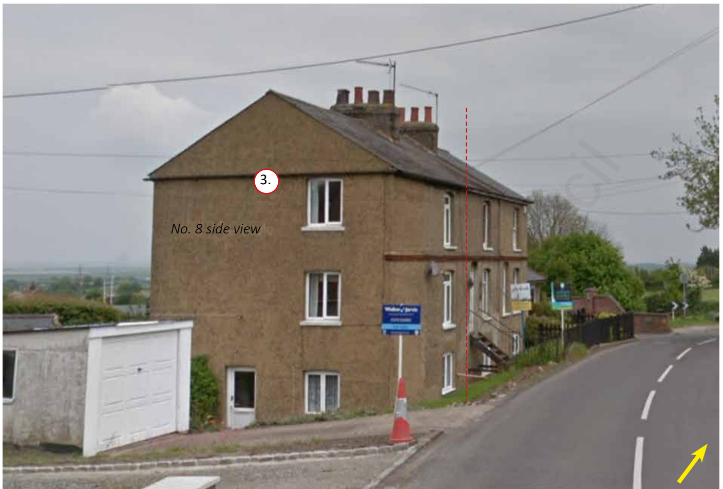
Heading out of village along Forge Lane looking to row of terraces to left
