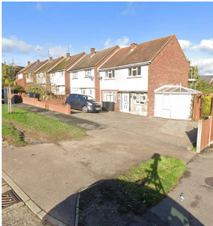
Photo of the existing dropped kerb at no. 60 Livingstone Road
