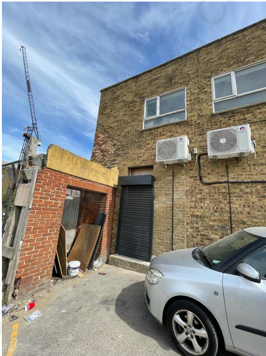
Picture 1.2.1 Visited point 1 - Back yard of all proper
