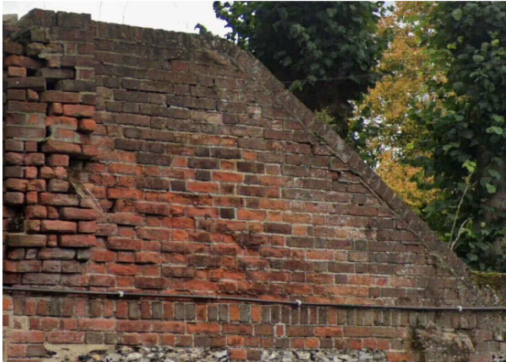
Reconstructed brickwork to match existing parapet wall bonding and mortar. 3 brick corbel to also be reinstated
