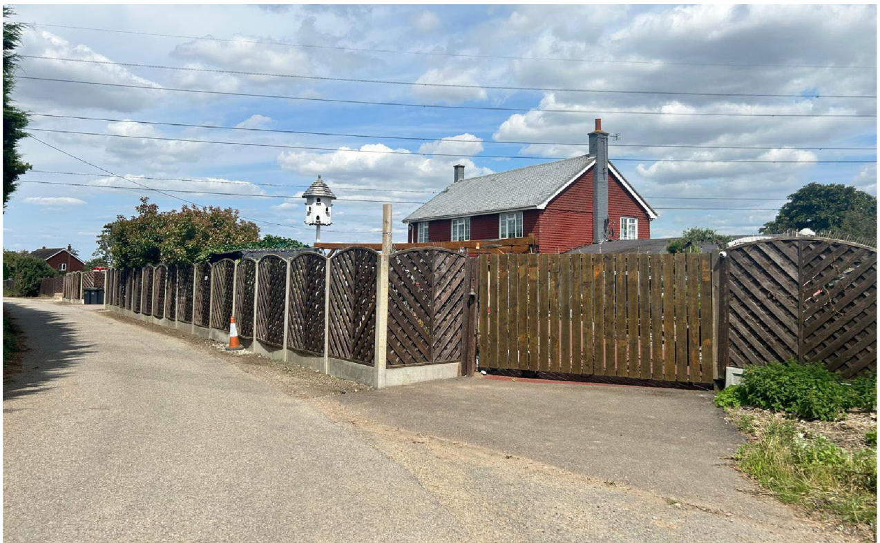
Figure 2a: Photograph looking northwards along Northfleet Green Road, showing front boundary and corner view of Dawes Cottage.
