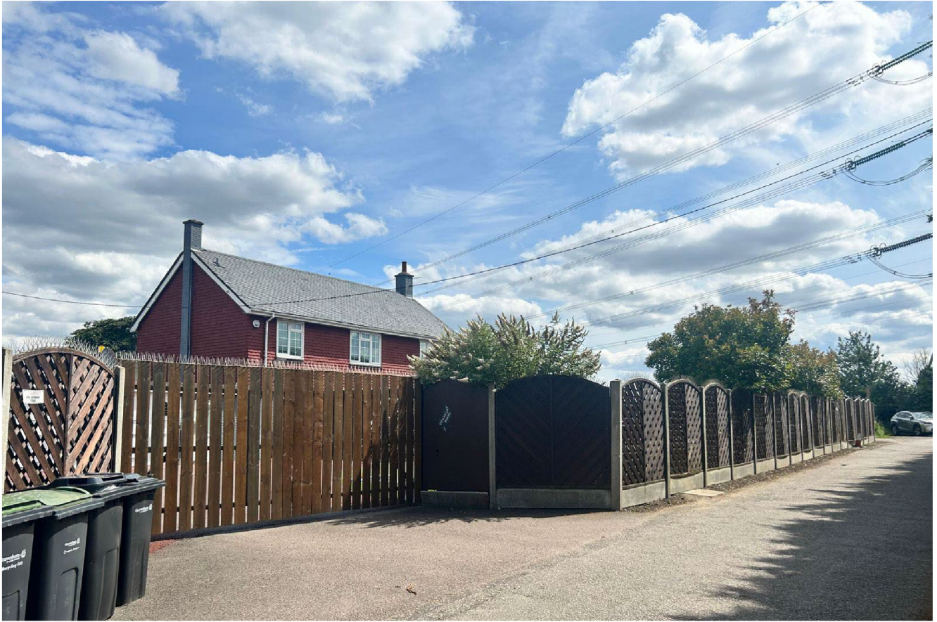
Figure 2b: Photograph looking southwards along Northfleet Green Road, showing front boundary and corner view of Dawes Cottage. Pylon visible on right side of image with overhead wires crossing the site to the south side of the main dwelling.
