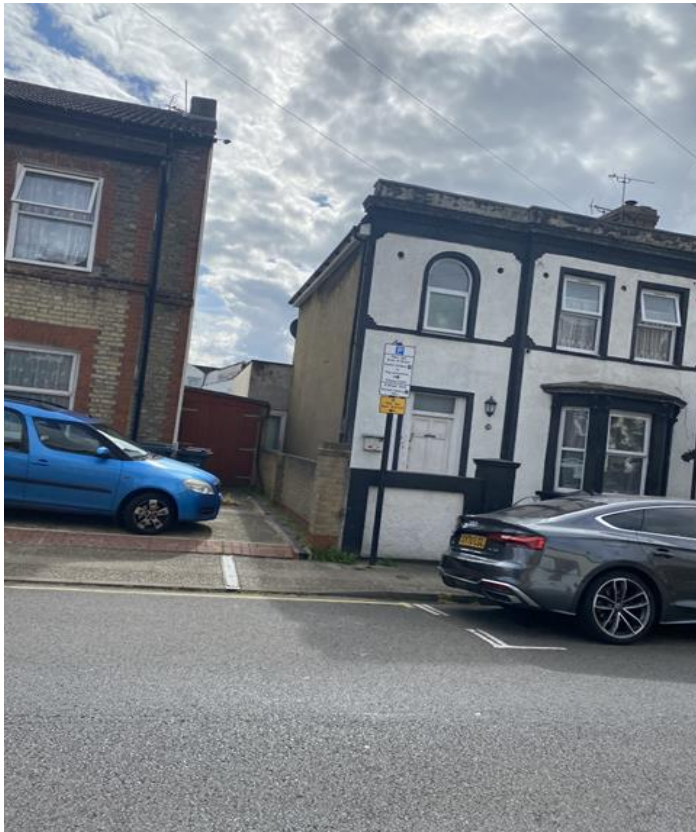
Garage & single storey extensions at 24 & 25 Darnley Street
