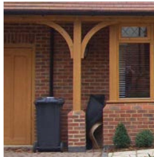
Facing bricks - Red multi Butterley Red Bank Coronet. Mortar colour to match brick. Oak timber posts
