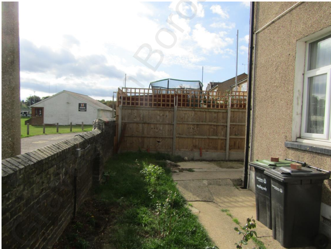
View across east facing frontage of Rose Cottage to garden of adjoining property to the south
