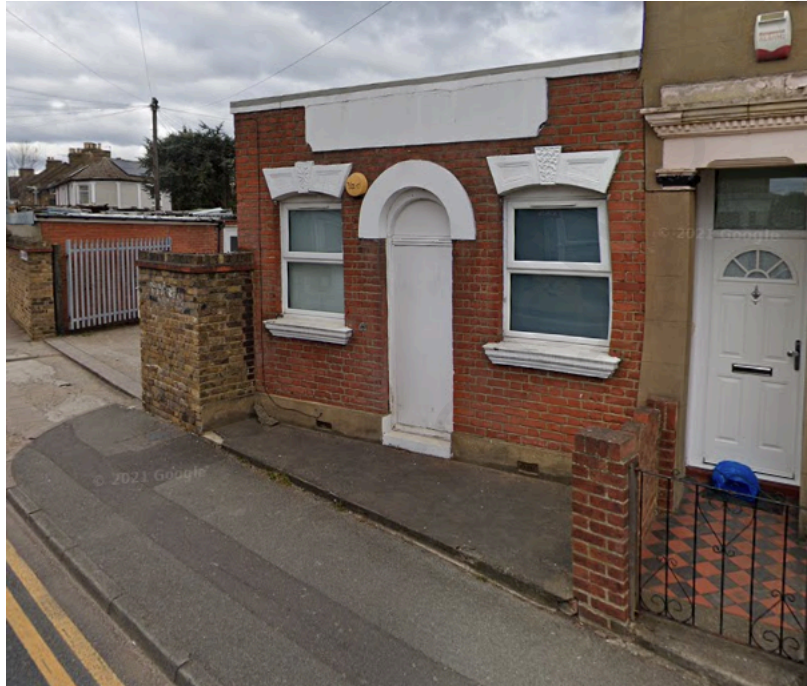
Image Six: Single storey brick building 25 metres to the south of the site (52 Dover Road East)
