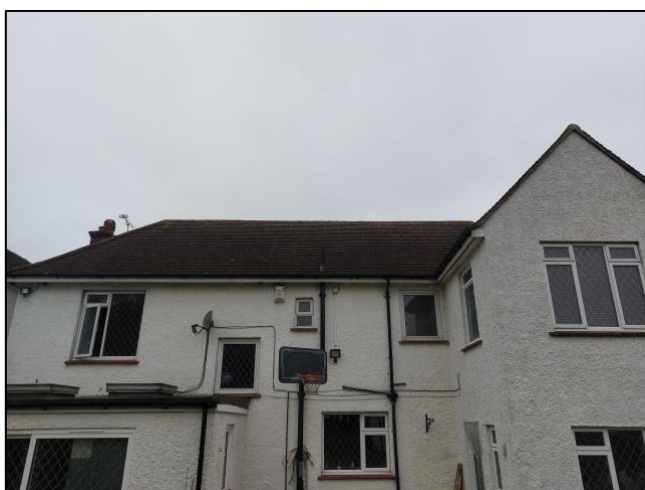
Photograph 1. Overview of the rear elevation.
