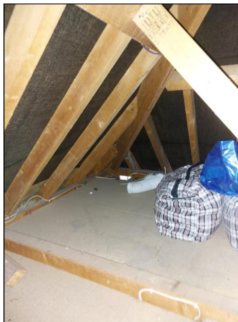
Photograph 10. Internal loft void.
