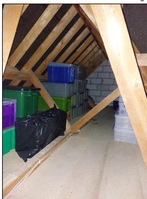
Photograph 8. Internal loft void.
