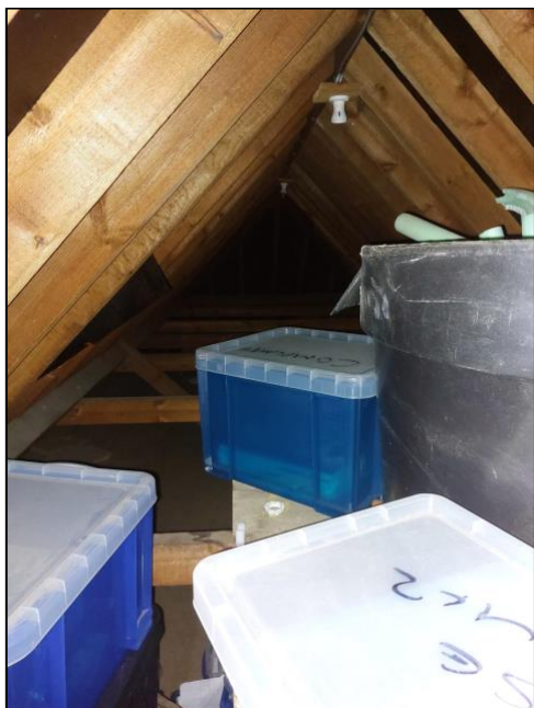
Photograph 9. Internal loft void.
