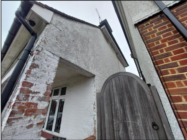
Photograph 12. Side (southern) elevation, note chimney that could not be fully viewed.
