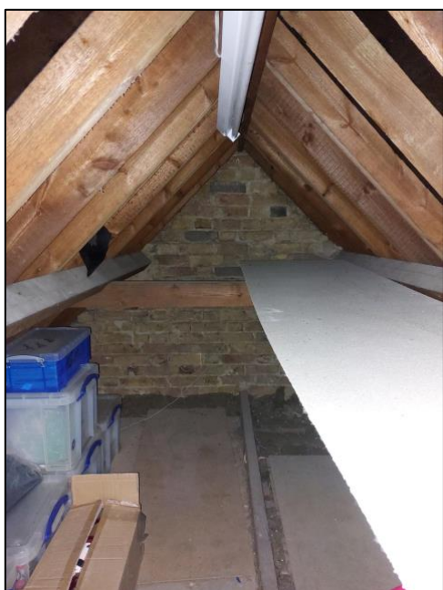
Photograph 11. Internal loft void.
