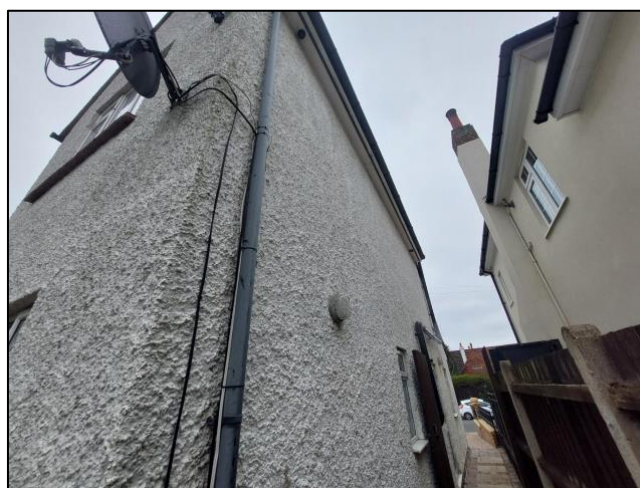
Photograph 12. Side (northern) elevation.
