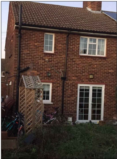
REAR ELEVATION PHOTO
