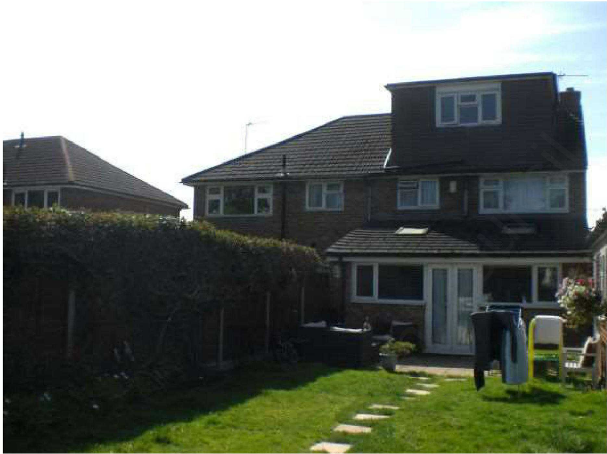
Looking towards the rear of 20 Vigilant Way (on left hand side)
