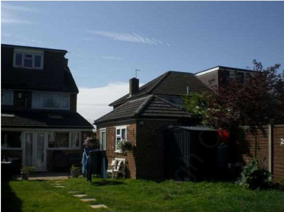
Looking towards the rear of 24 Vigilant Way (on right hand side)
