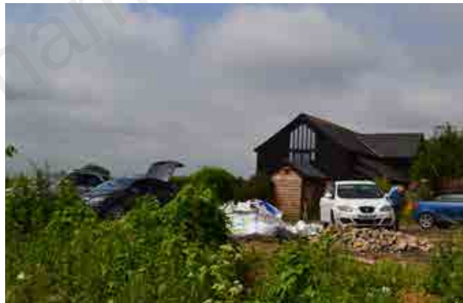
The site is used as a yard for storage of materials, vehicles and plant and detracts from the setting of the residential barn and farm buildings. The boundary vegetation is weak on the eastern side of the yard where it slopes down to the arable fields
