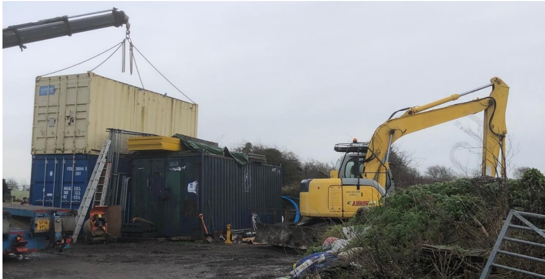
Figure 4 - Photo on site showing double stacked containers
