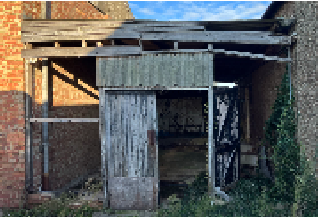
looking at the south elevation from outside
