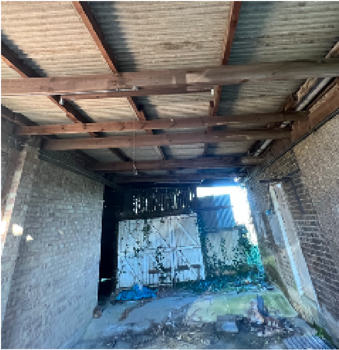
looking at the north elevation from inside
