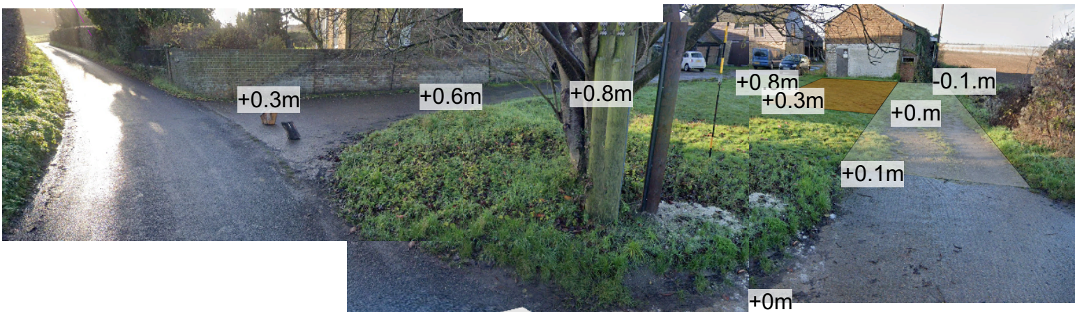
view of existing site access - showing levels using the edge of the road at the access point as a datum
