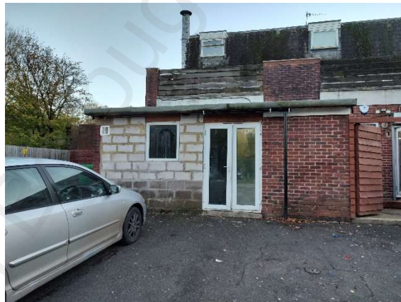
Fig 4. Photo to the rear
