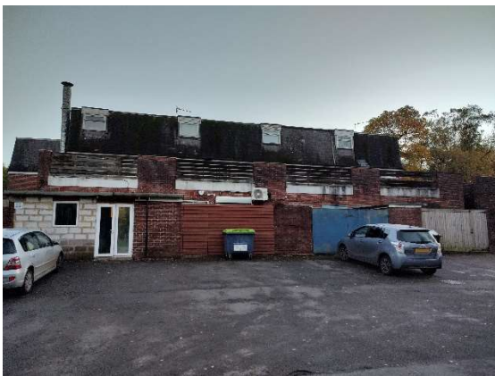
Fig 3. Photo to the rear
