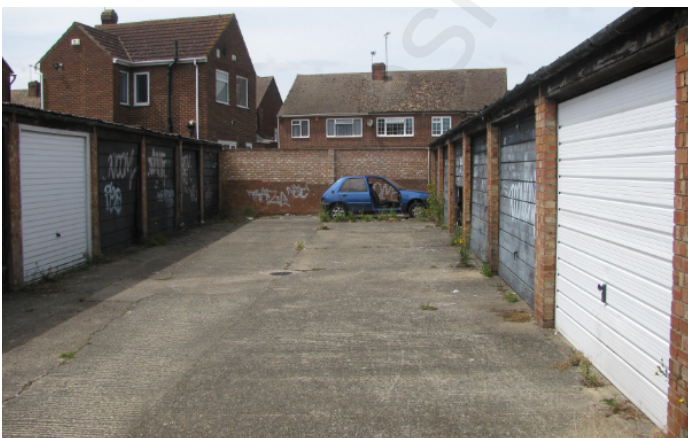
Inside the existing garage court
