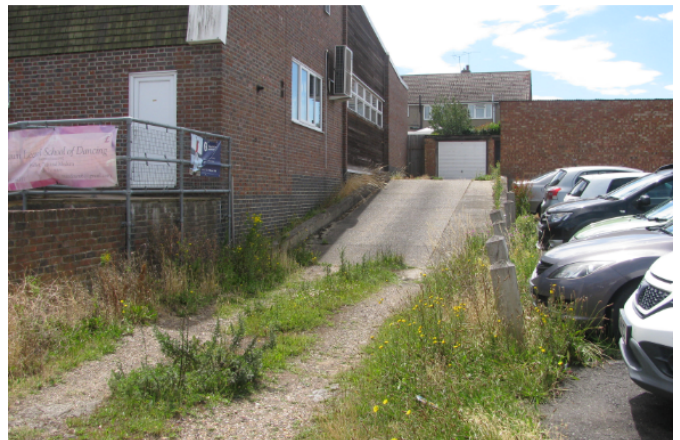
Ramped access to the garage court
