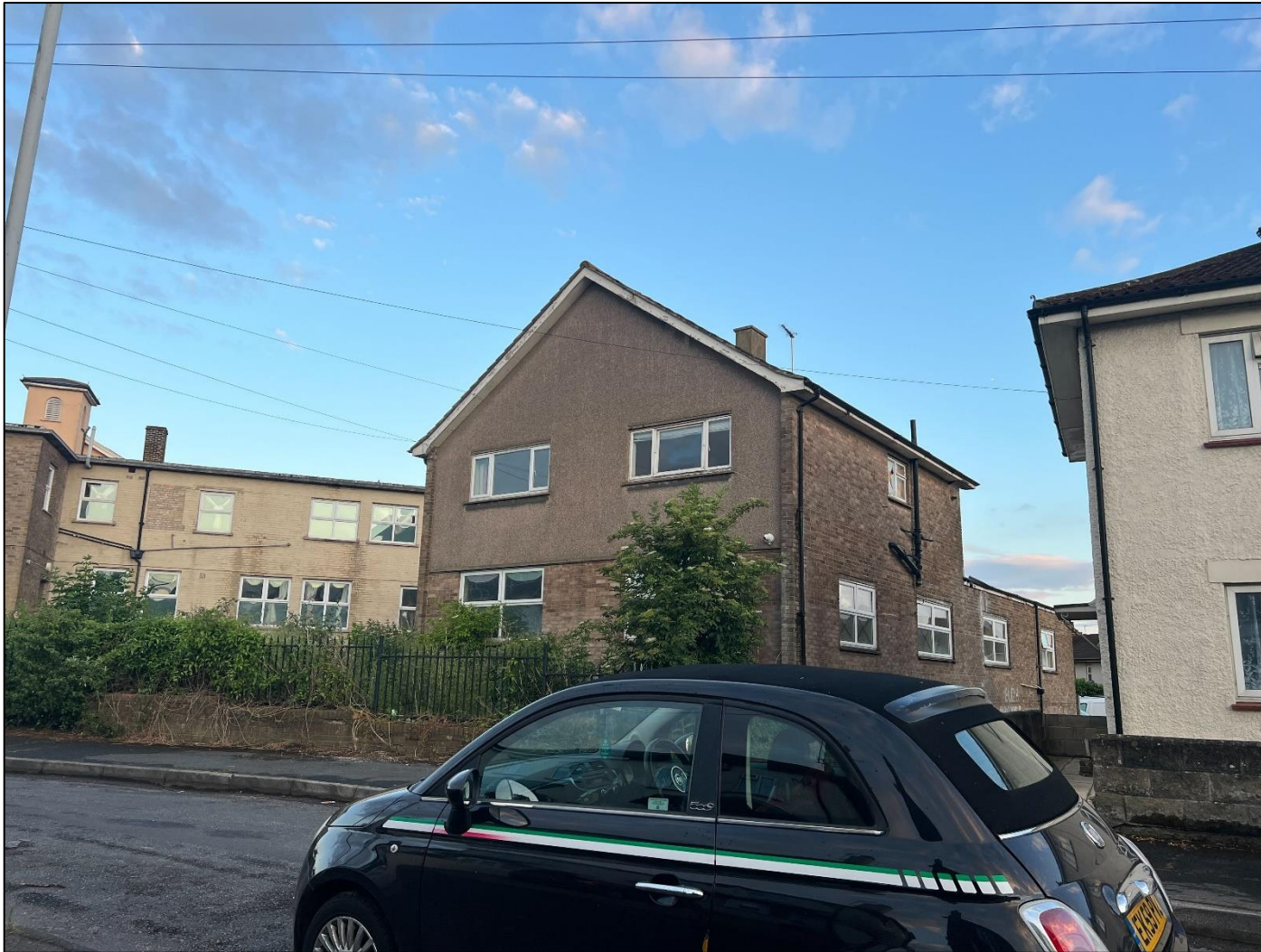
Photo 1: The northern elevation of B1 before the survey on 10/06/2024
