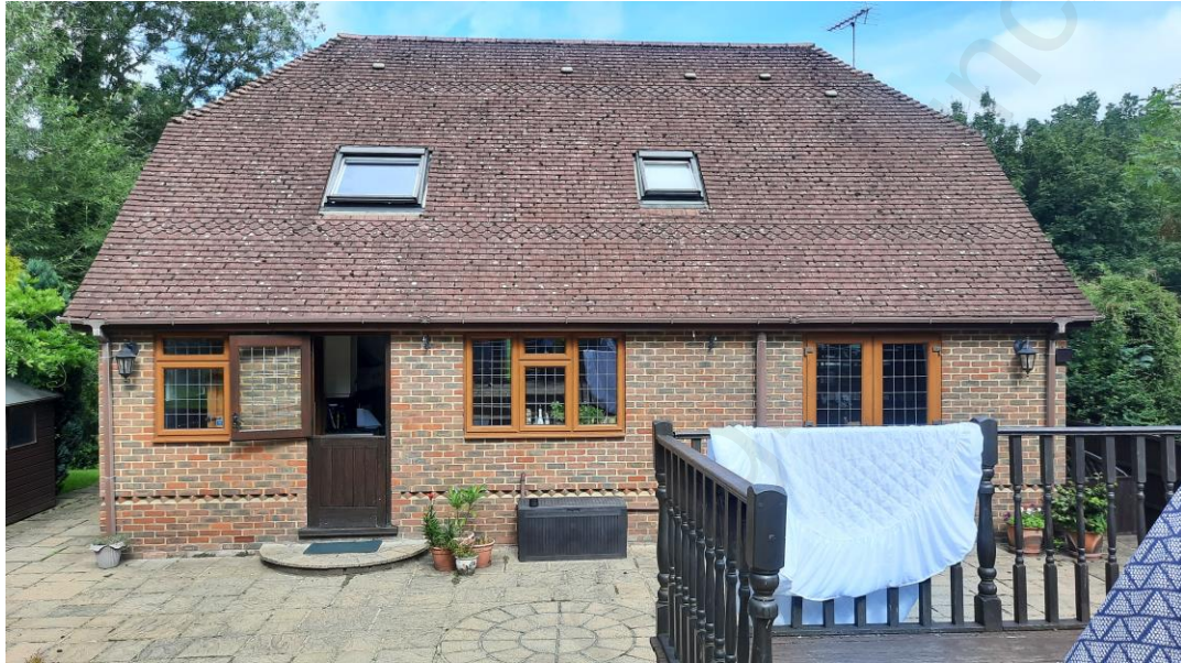
Photograph 1: Existing rear elevation
