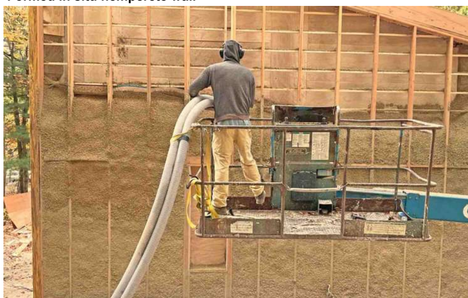
Formed in situ hempcrete wall
