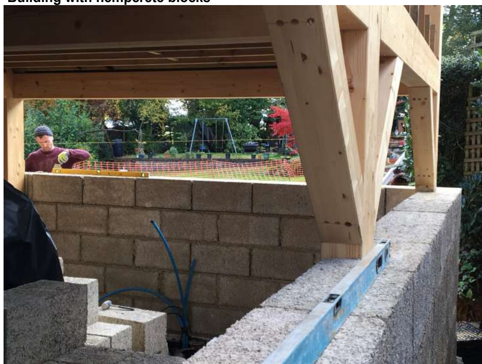
Building with hempcrete blocks
