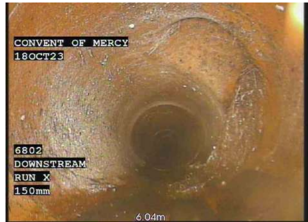
2, 00:01:13, 6.04 m Roots, mass, 5% cross-sectional area loss
