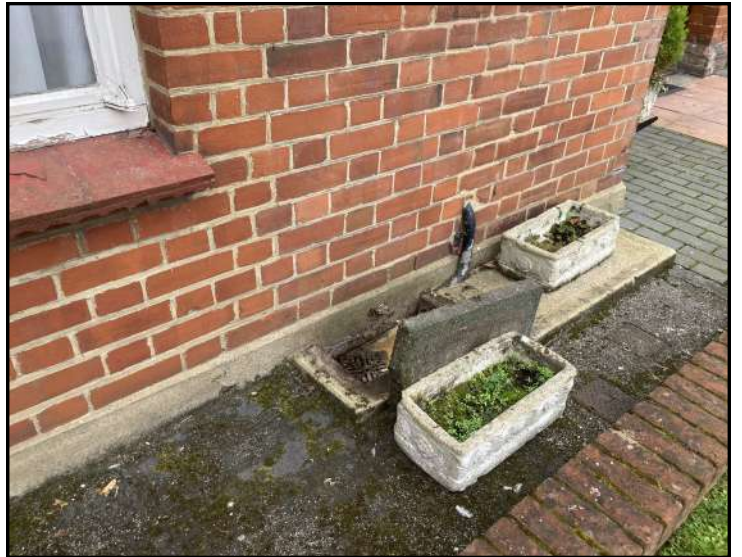
LOCATION OF FOUL GULLY 2
