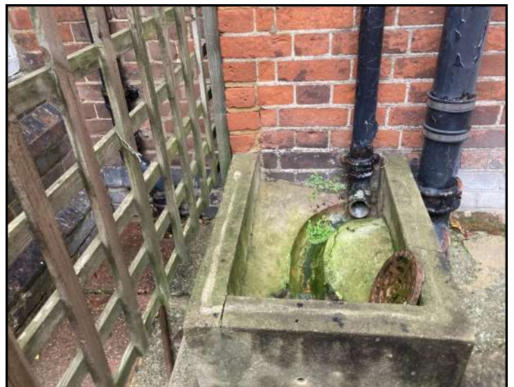
LOCATION OF FOUL GULLY 4
