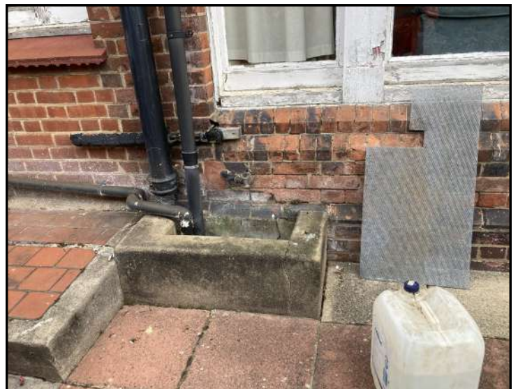
LOCATION OF FOUL GULLY 1
