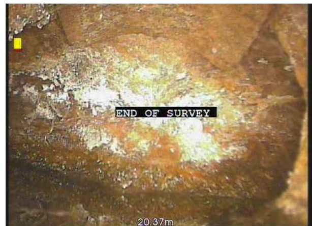
4, 00:03:36, 20.37 m Finish node, outfall, reference: IC4-A, At Y junction - unable to continue
