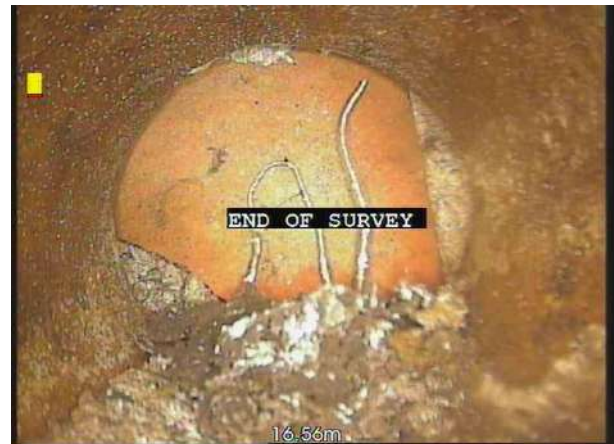
2, 00:02:30, 16.56 m Finish node, outfall, reference: IC4-B, At capped / redundant end
