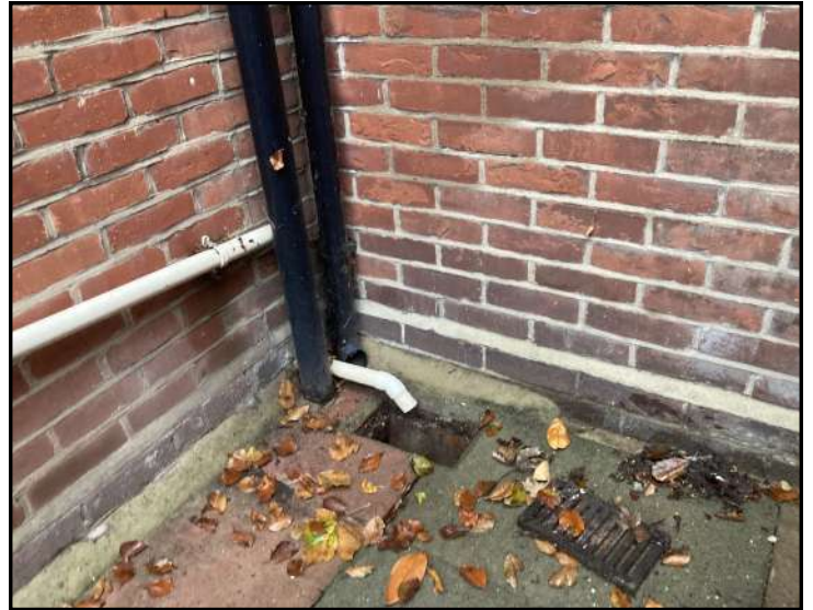
LOCATION OF COMBINED GULLY 5
