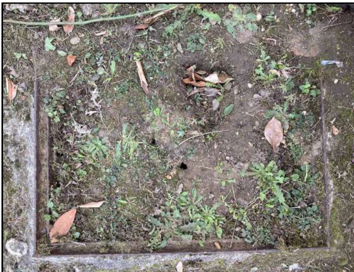
MH1. CHAMBER FILLED IN
