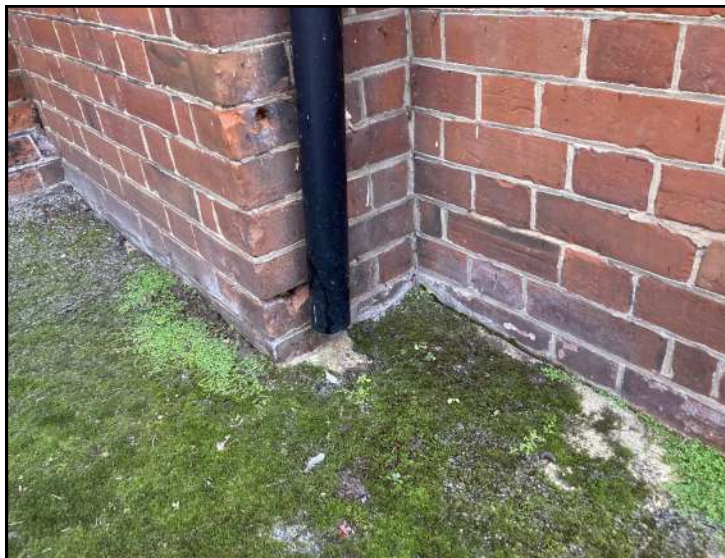
RWP 1. INTO GROUND
