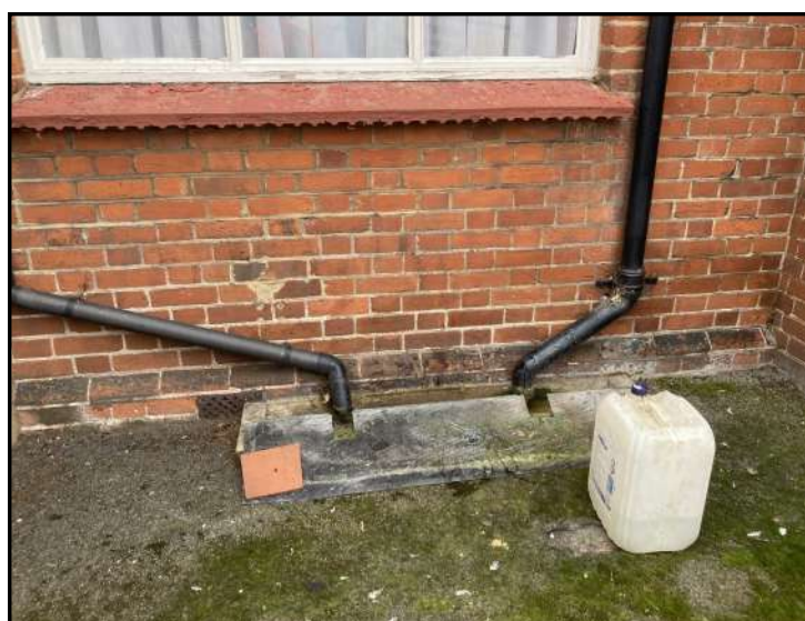
LOCATION OF COMBINED GULLY 3
