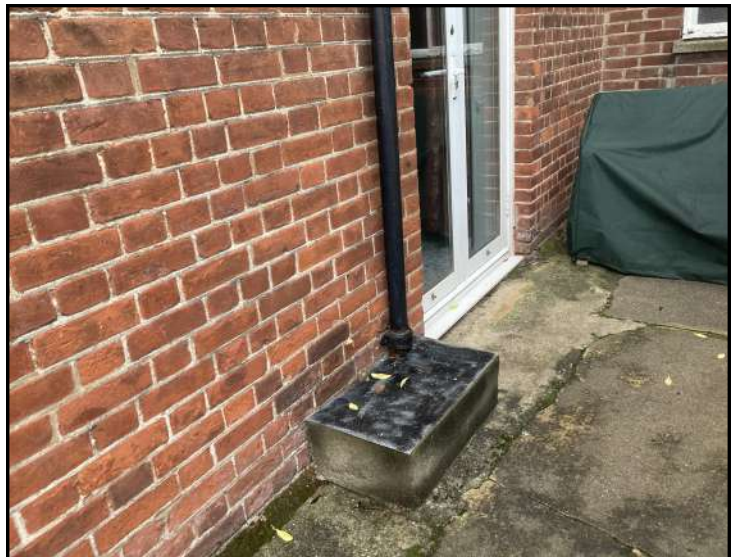
LOCATION OF FOUL GULLY 5
