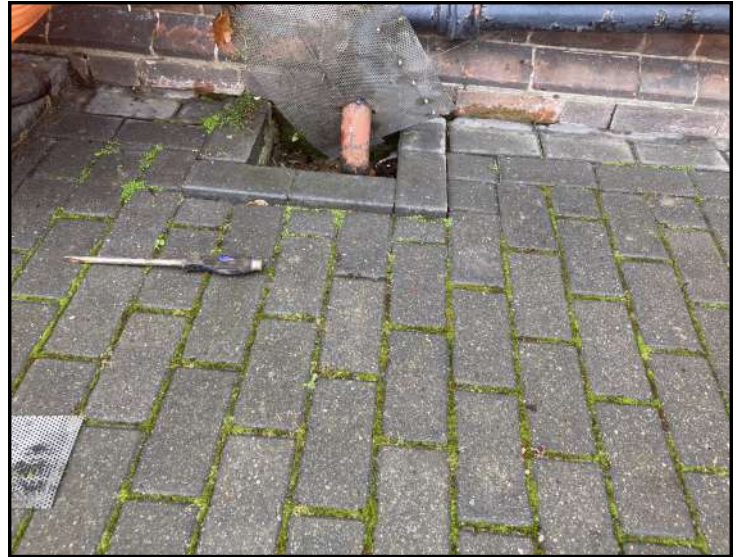
LOCATION OF FOUL GULLY 3
