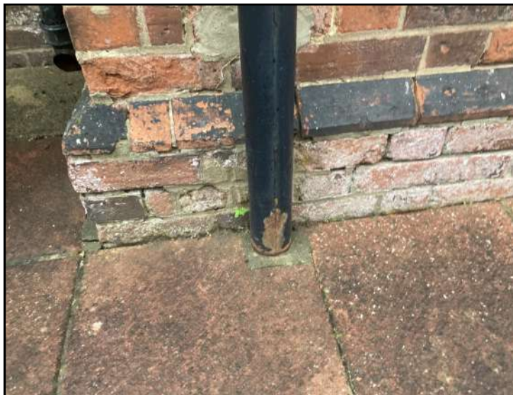
RWP 4. INTO GROUND
