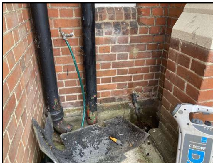
LOCATION OF COMBINED GULLY 2
