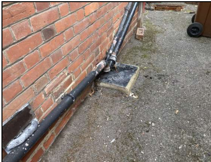
LOCATION OF COMBINED GULLY 4
