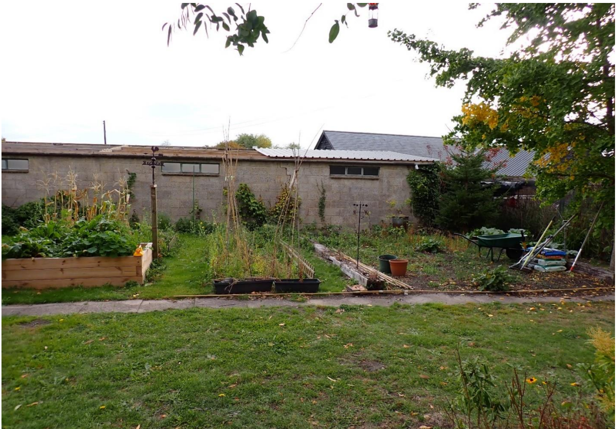
Photo 16. Southern boundary building.
