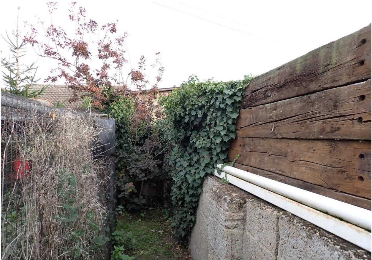
Photo 25. Southern boundary block and sleeper wall.
