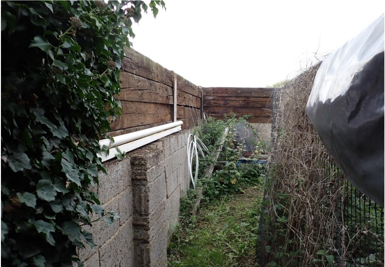
Photo 21. Southern and western boundaries block and sleeper wall.
