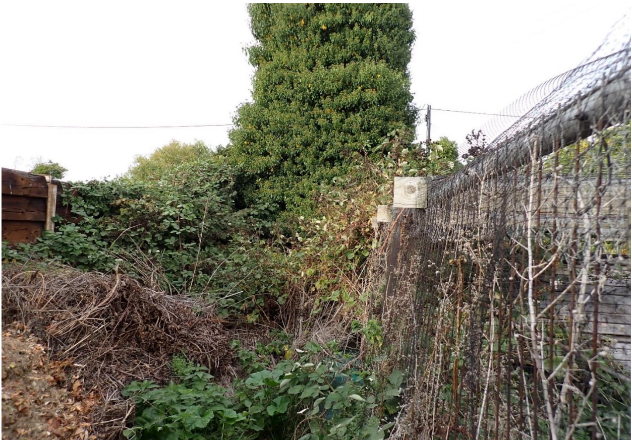
Photo 24. Western boundary block and sleeper wall.
