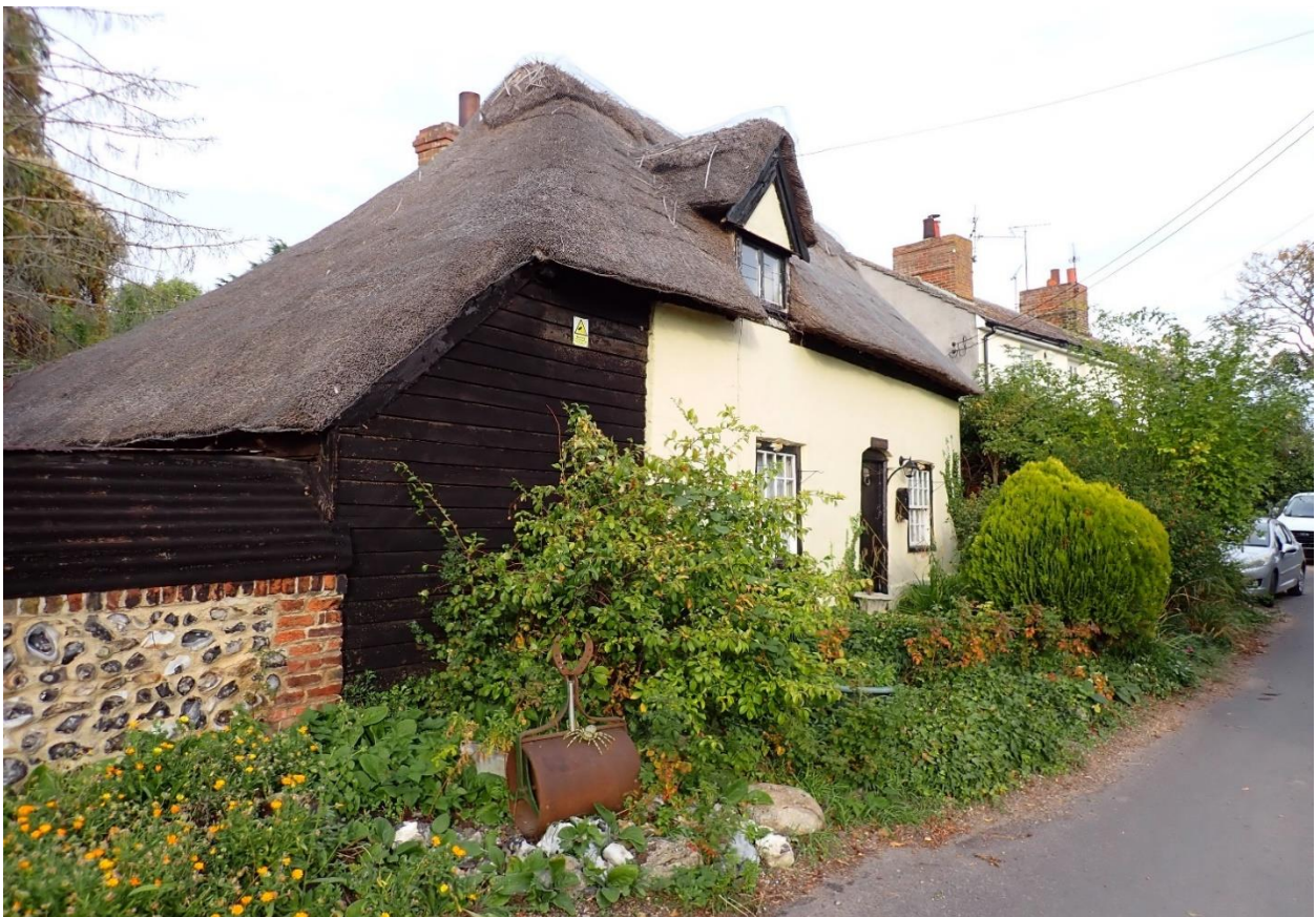
Photo 6. Clerk's Cottage, Church Street.
