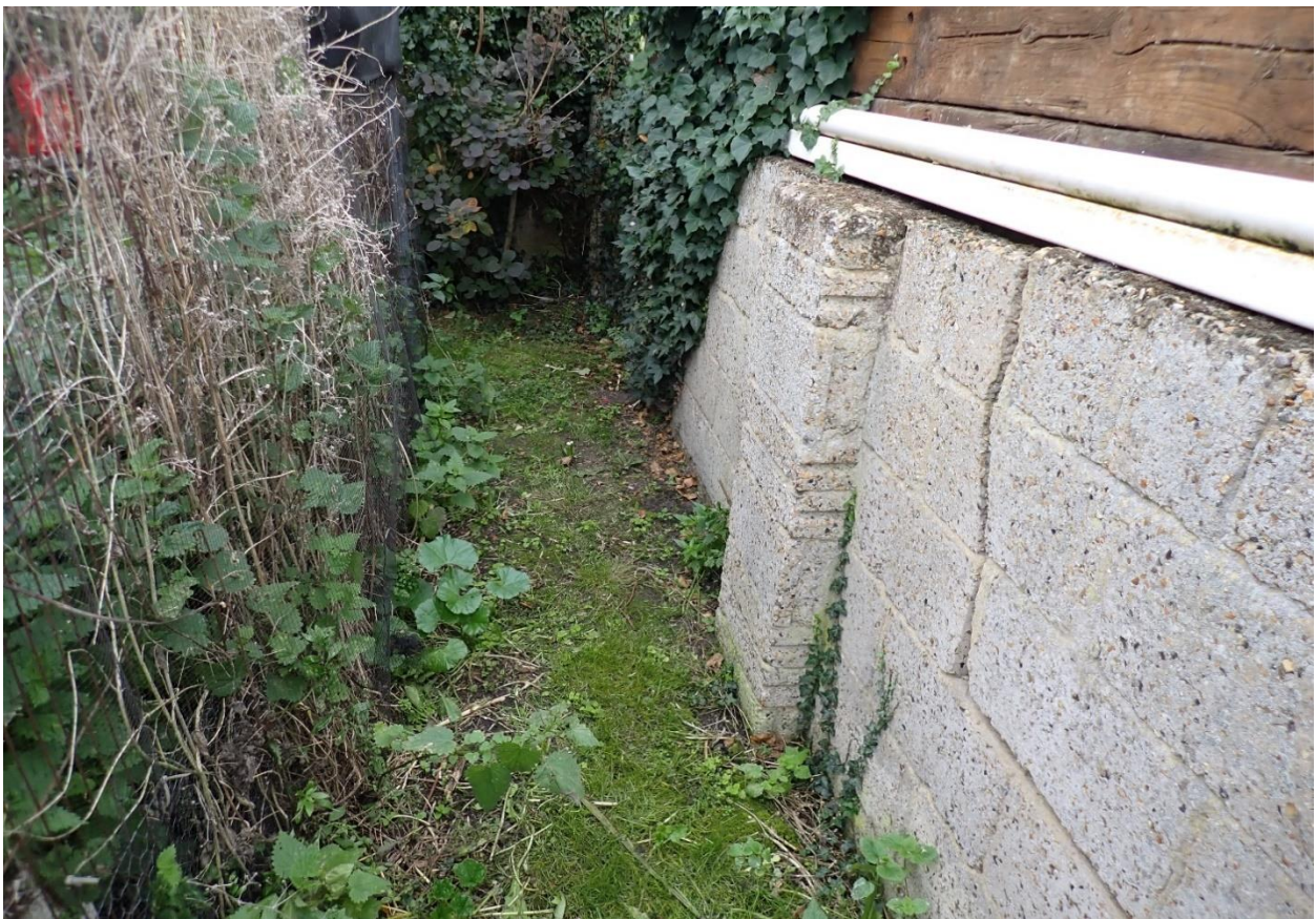
Photo 26. Southern boundary block and sleeper wall.
