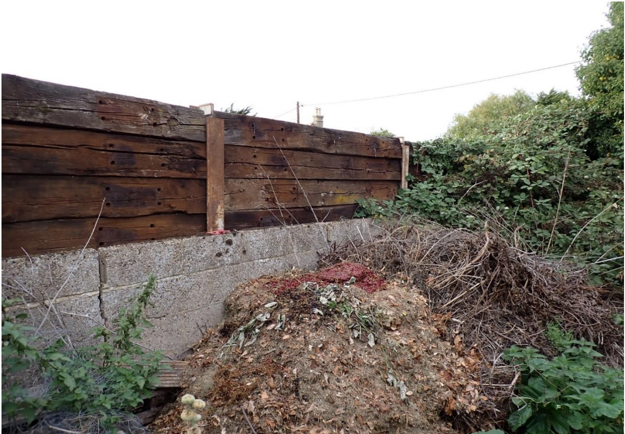
Photo 23. Western boundary block and sleeper wall.
