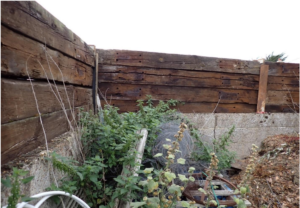
Photo 22. Southern and western boundaries block and sleeper wall.
