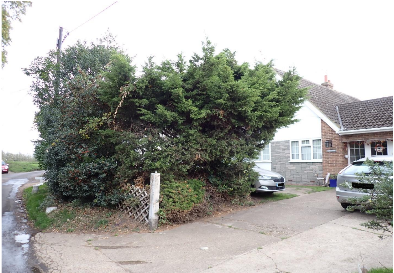
Photo 1. Front elevation of Farmcroft.
