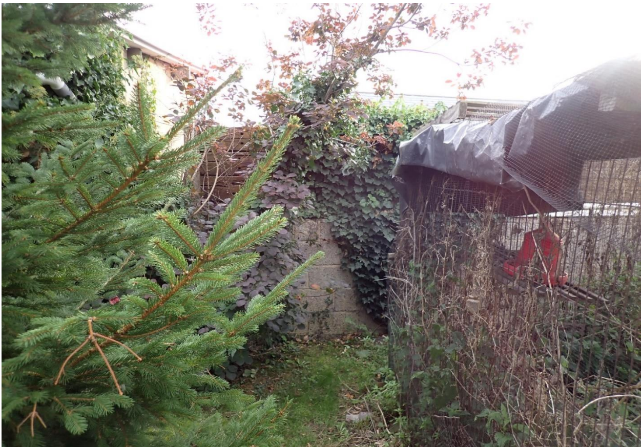
Photo 20. Southern boundary block and sleeper wall.
