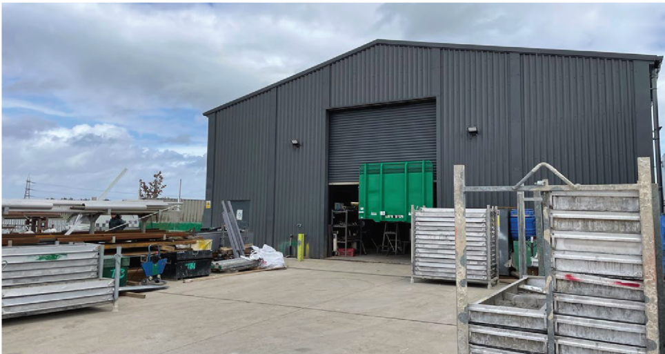
An additional storage building
