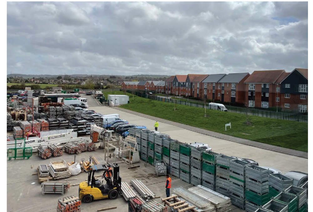
The external storage area on the east side of the site, with the three storey housing on the opposite side of Dalefield Way visible beyond the access road and the bund.
