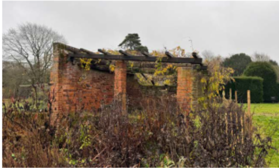
2. View of north west elevation of Loggia
