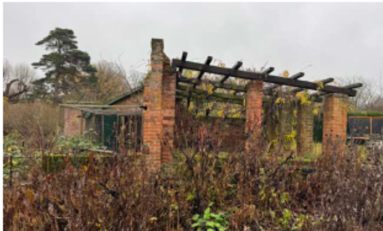
3. View of north west elevation of Loggia and Potting shed
