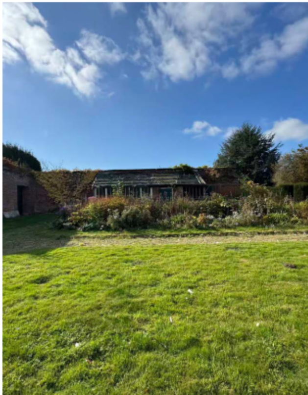
1. North elevation of potting shed
