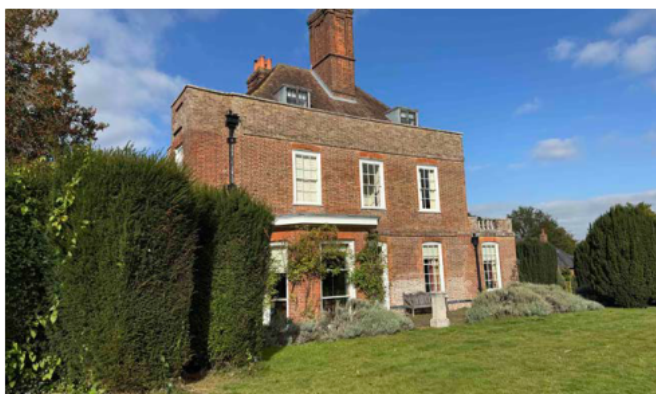
1. South-eastern elevation showing affected gutter outlet
