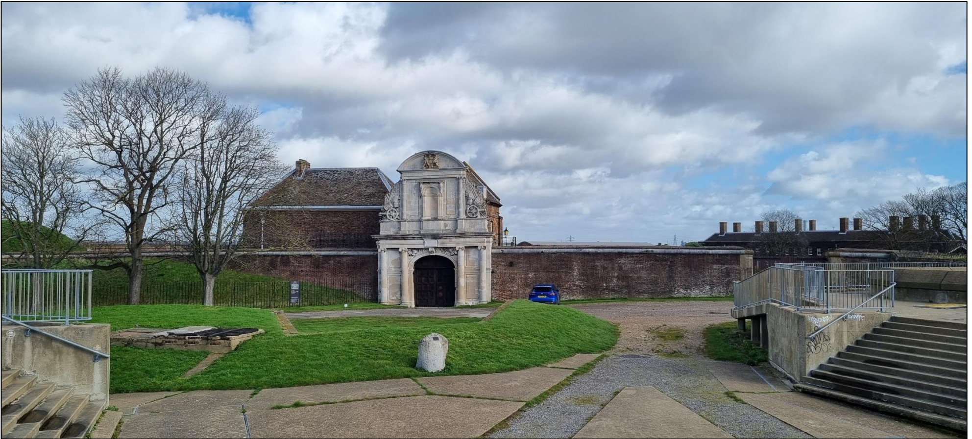
Plate 1: Tilbury Fort gatehouse looking north.
