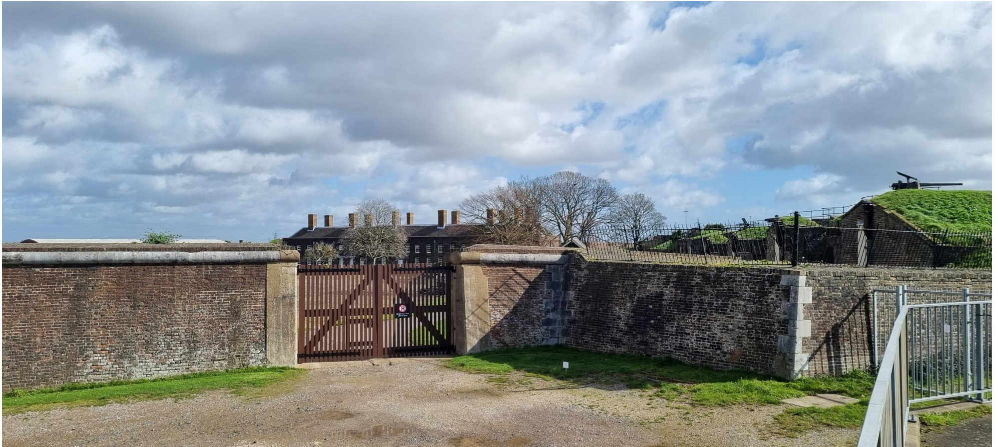
Plate 2: The grade II* listed Officers Barracks within Tilbury Fort, looking northeast.
