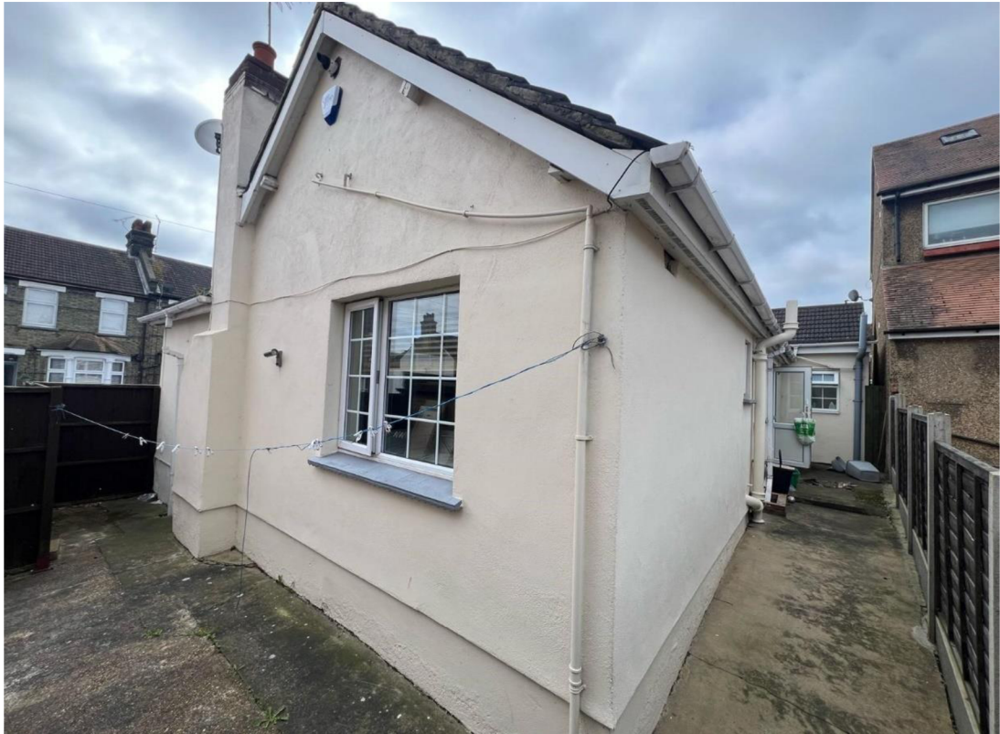
Image 4: Photo of north and west (rear) elevations of property from northwestern corner of site demonstrating the hardstanding nature of the existing residential curtilage.
