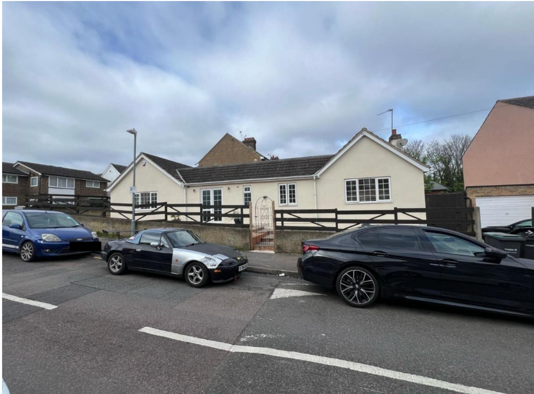
Image 2: Photo of east elevation of site from Russell Road
