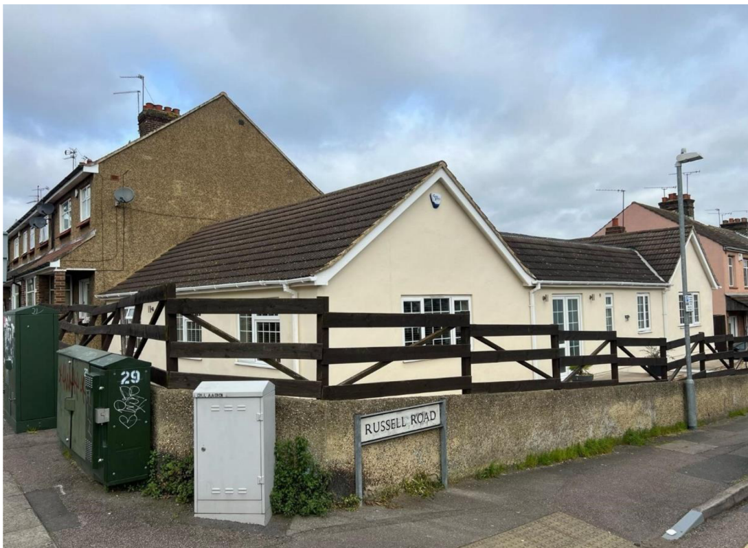
Image 3: Photo of eastern and southern elevations of site as seen from corner of Russell Road and Albion Terrace. This image demonstrates how the existing property does not relate to the height/scale of the neighboring terraces.
