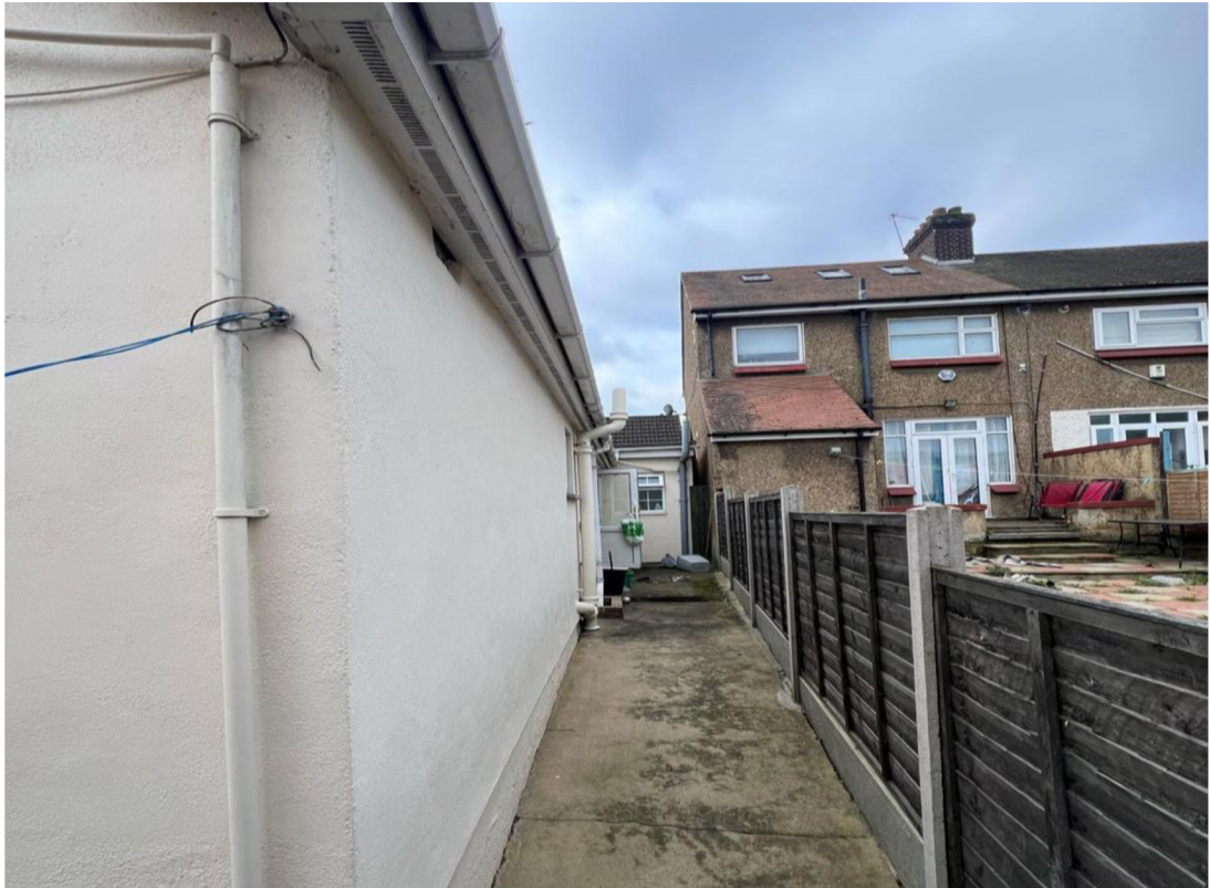
Image 6: Photo of existing western boundary with rear elevation of No 25 Albion Terrace visible in background
