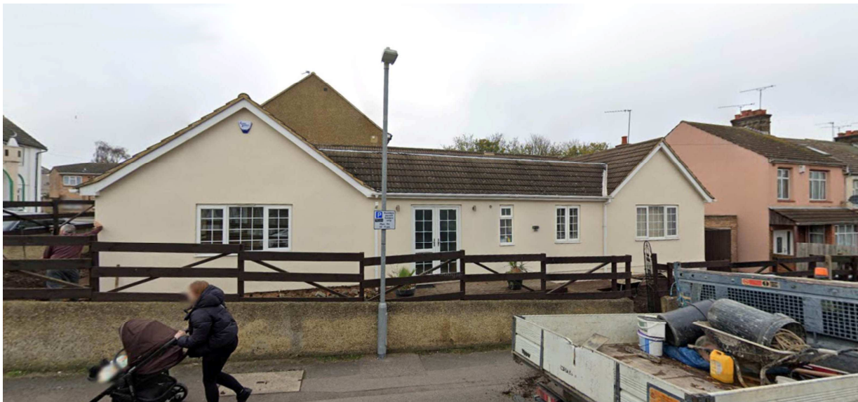
Existing bungalow viewed from Russell Road
