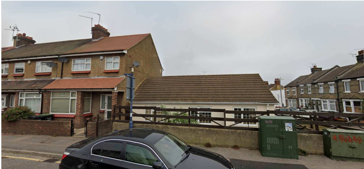
Existing bungalow viewed from Albion Terrace
