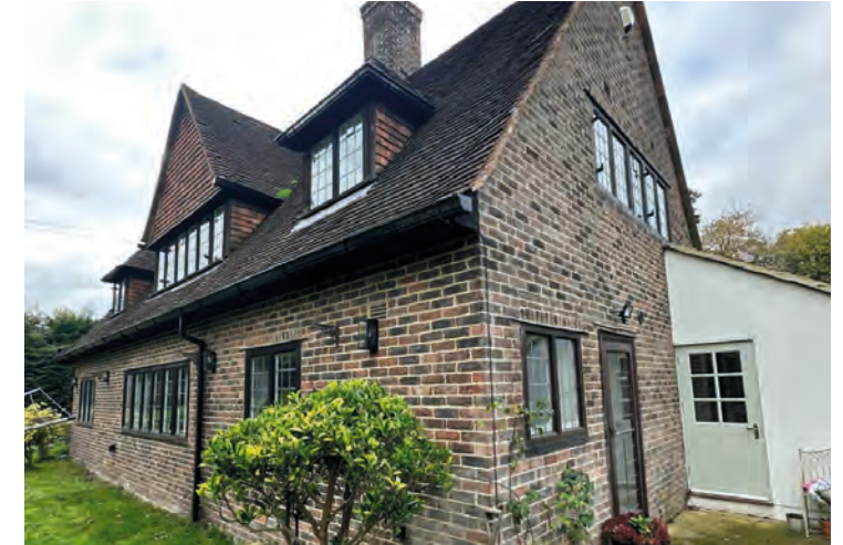
Image 4: This image shows the North Eastern elevation of the existing building.
