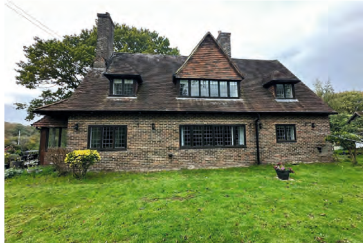
Image 1: This image shows the elevation fronting Pear Tree Lane which the previous Prior Approval application confirmed at the principle (front) elevation.
