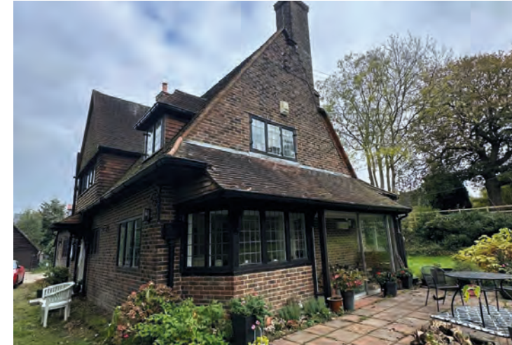
Image 3: This image shows the South Western elevation of the existing building.
