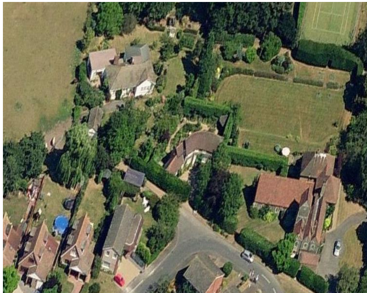
P001 – aerial view of site looking westerly
