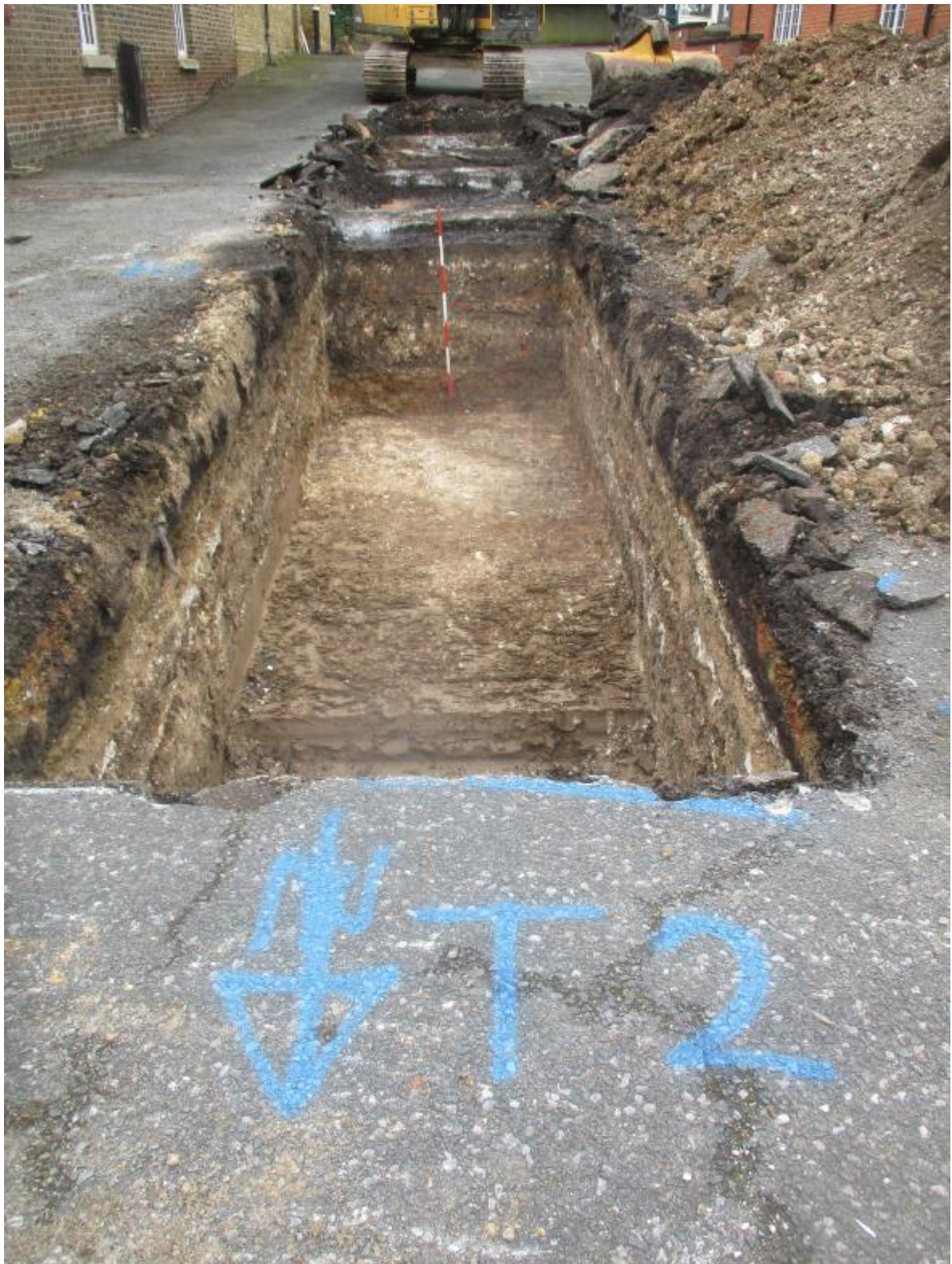
Plate 15. Trench 2 (north-south aligned and cut at a right angle some 3m south of and perpendicular to Trench 1), looking south with natural orange-brown brickearth underlying a 1.2m-thick layer of made ground (1.4m scale)
