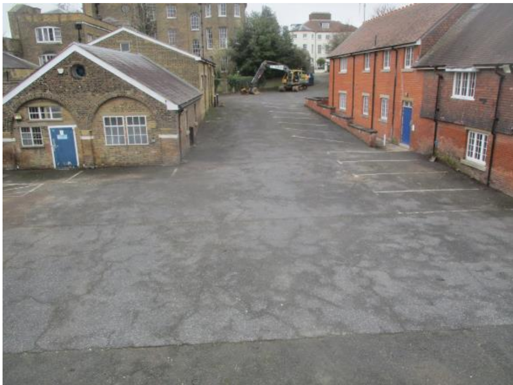
Plate 4. The boathouse looking south with red-brick ancillary buildings to the right (west)
