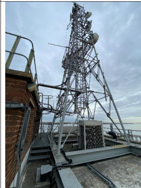
Figure 13 Mast to be relocated on the roof of B3.
