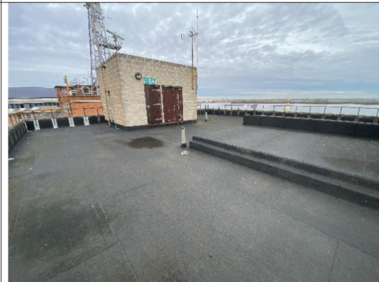
Figure 19 Roof of B5.
