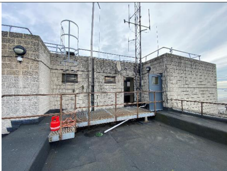
Figure 20 Roof of B5
