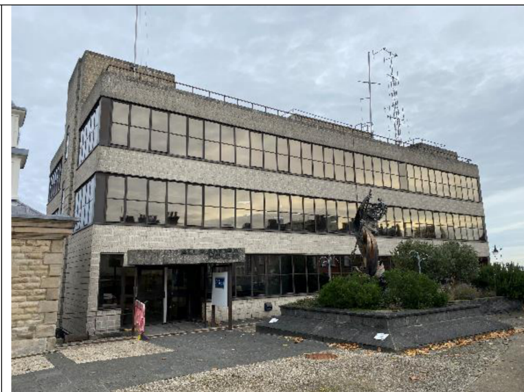
Figure 17 Southern and western elevation of B5.
