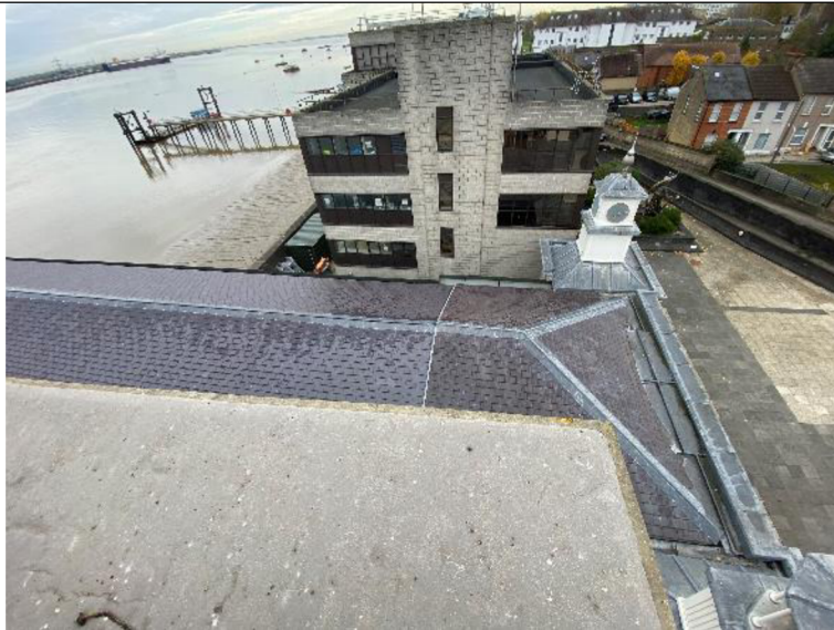
Figure 15 Roof of B4.
