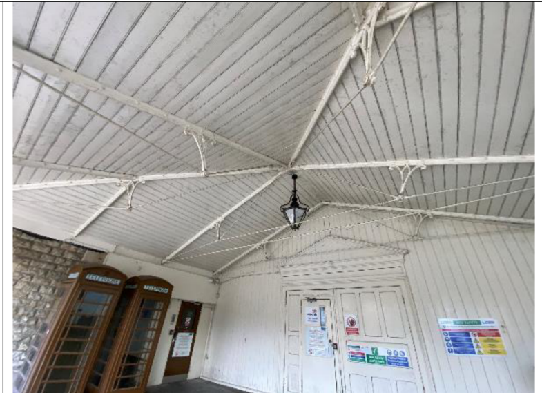
Figure 16 Interior of B4.
