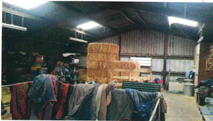
5. Internal above mezzanine level.
