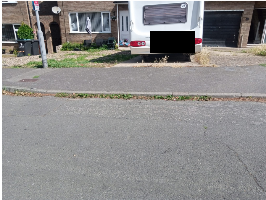
Photo showing the existing dropped kerb at 49 & 51 Nickleby Road
