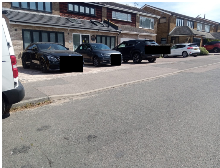
Photo showing a full length dropped kerb of 53 & 55 Nickleby Road
