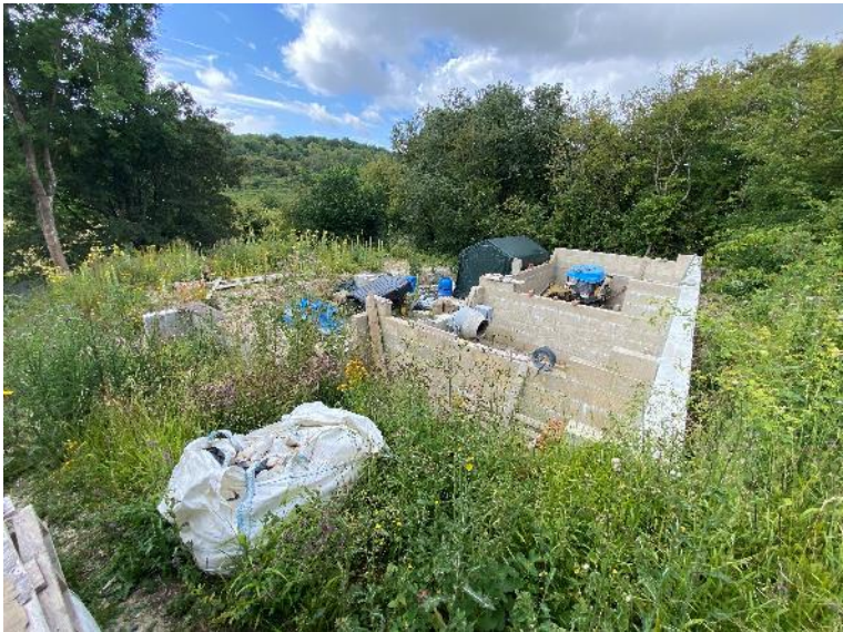
Figure 3 Existing hard standing area where the stable block will be built on.
