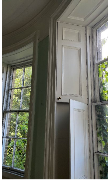
Examples of existing sash windows with timber shutters.
