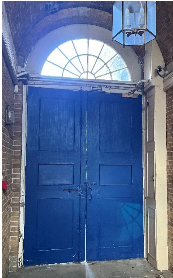
Main corridor door to rear inside.
