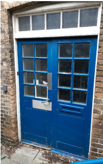
External door to unit 12.
