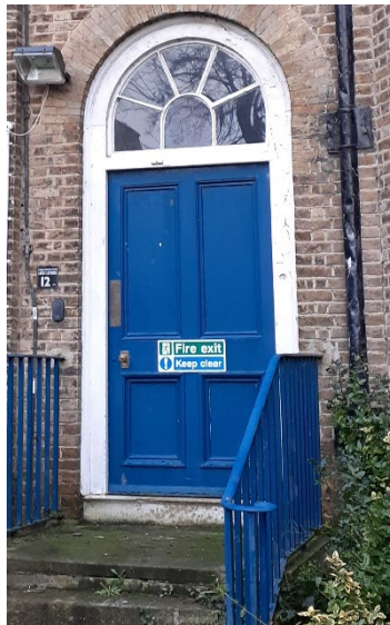
External door communal access point.
