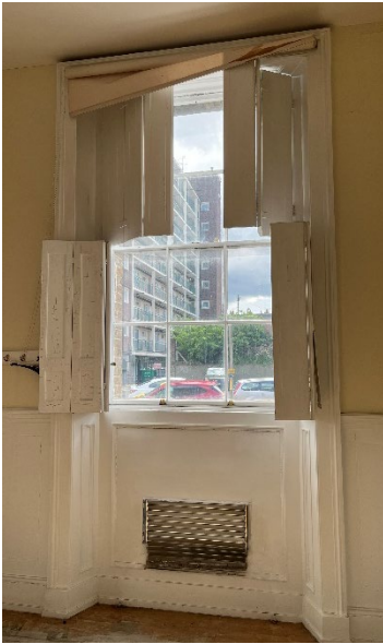
Examples of existing sash windows with timber shutters.
