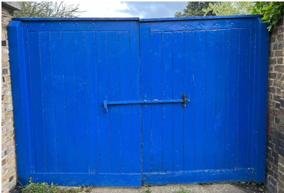
External view of double timber gates fronting The Terrace.
