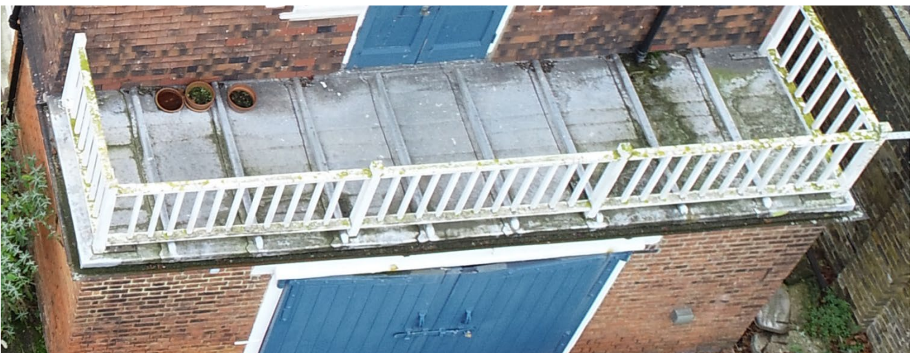
Lead floor finish to balcony.
