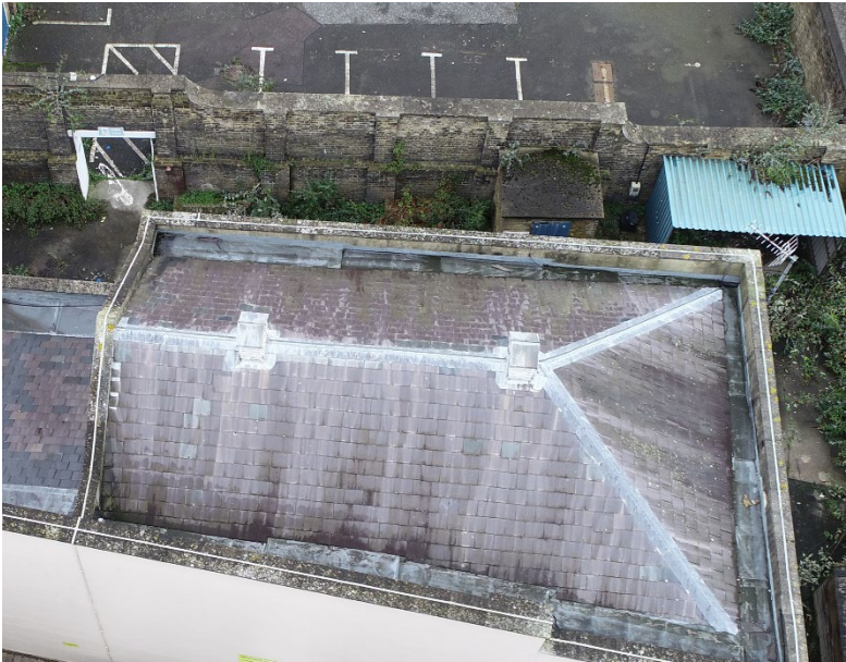
Outbuilding nearest the flood defence wall roof.
