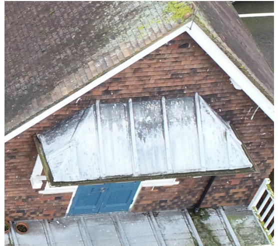
Lead roof over balcony.
