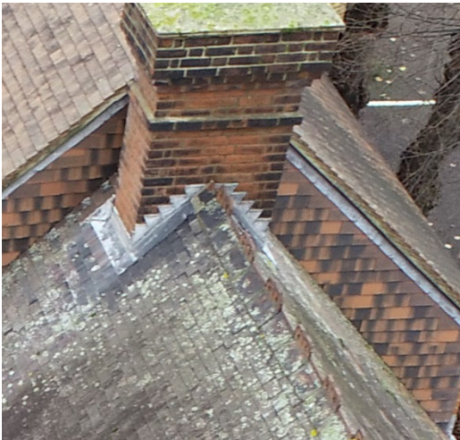
Lead flashing to chimney junction.
