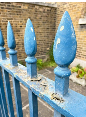
Images of railing corrosion and paint damage.
