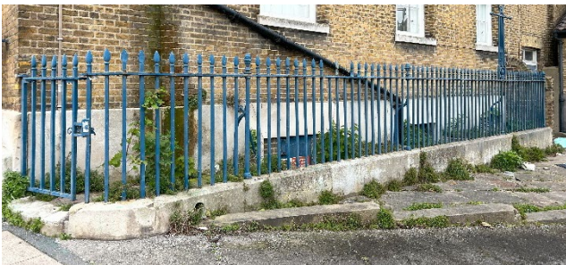
Main entrance railings 03 – Commercial Place.
