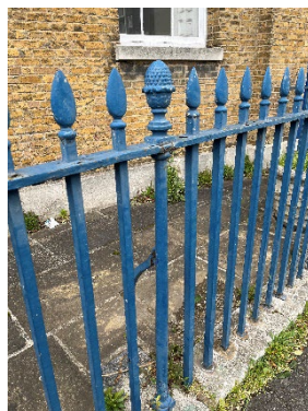
Images of railing corrosion and paint damage.
