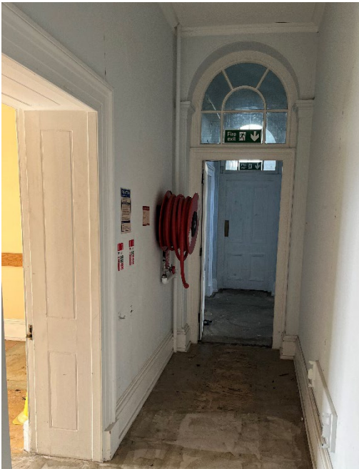
Examples of varying original architraves to be retained across the main house.
