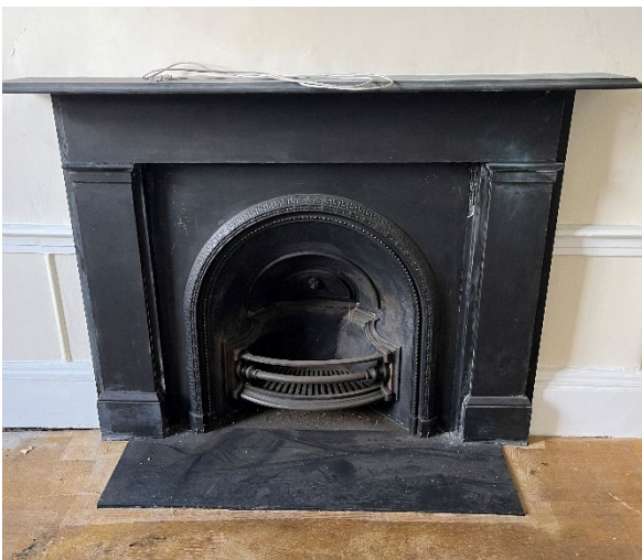
Front elevation to fireplace to Unit 6.
