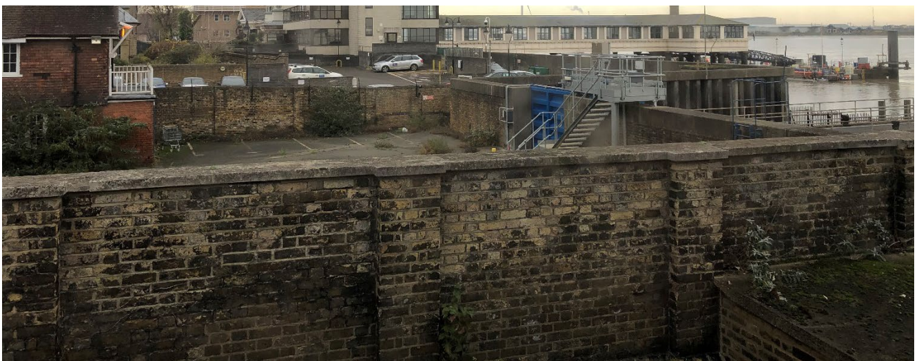
Image of stone coping to spine wall.
