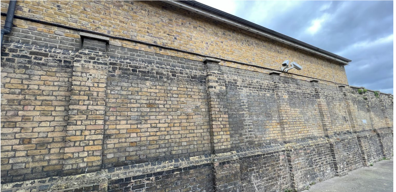
Image of existing workshop built off the spine wall. Clear delineation between existing spine wall and workshop building.
