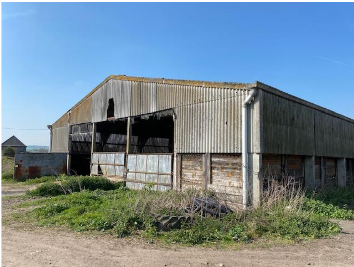
Existing Barn (Viewed from North East Elevation)
