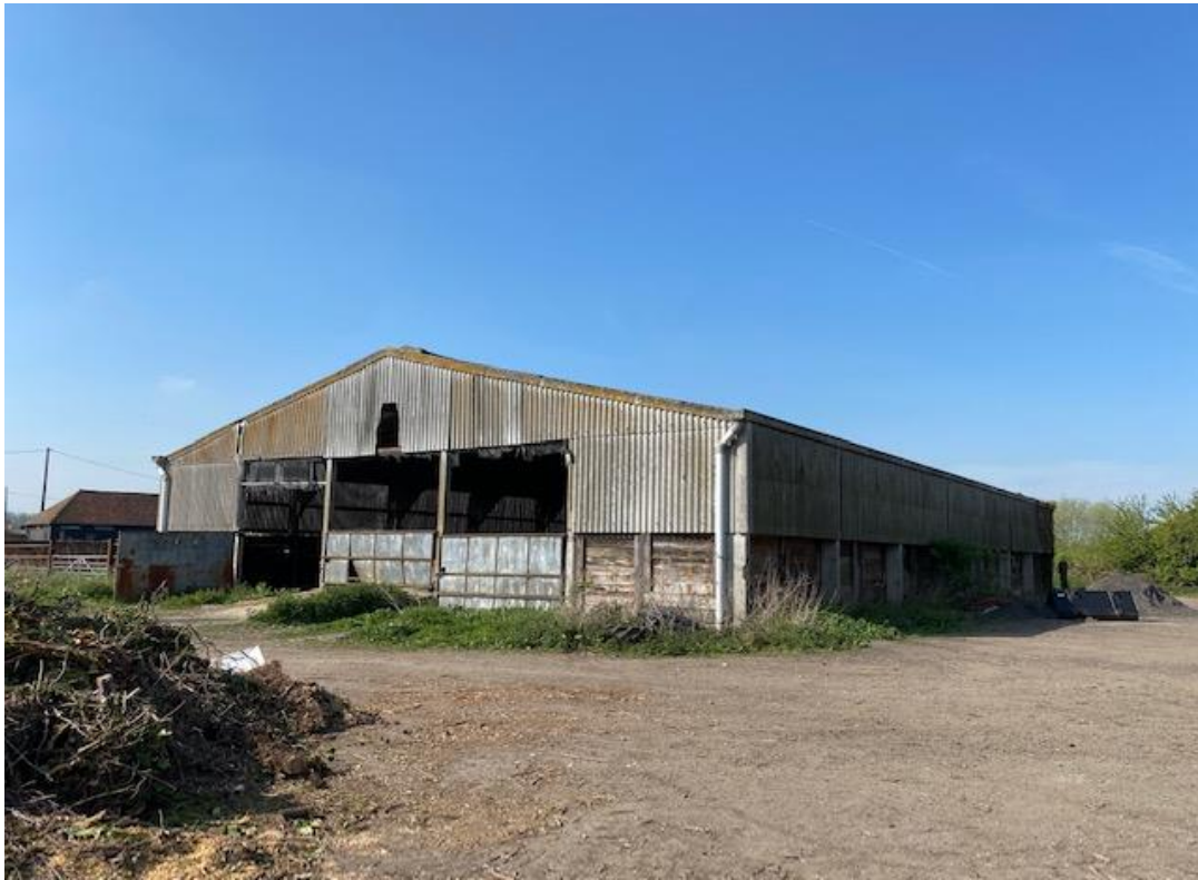
Existing Barn (Viewed from East)
