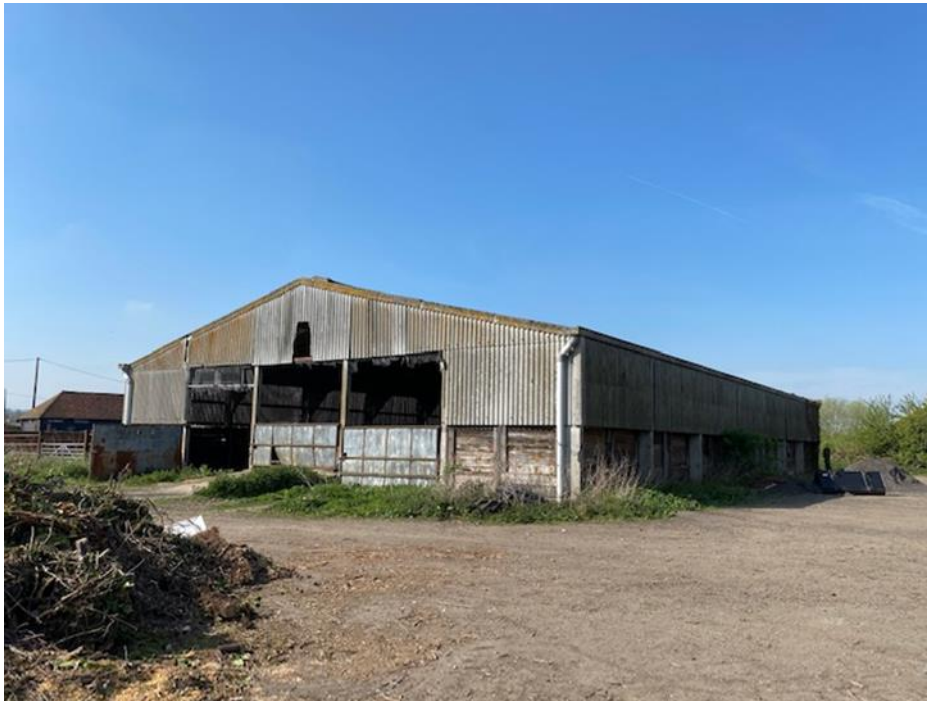
Photograph 1: Photograph of Existing Barn
