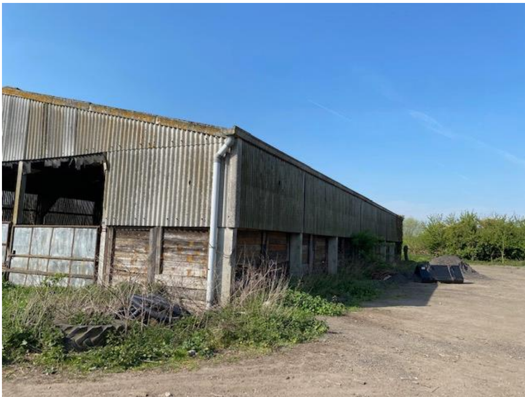
Existing Barn (Viewed from North Elevation)
