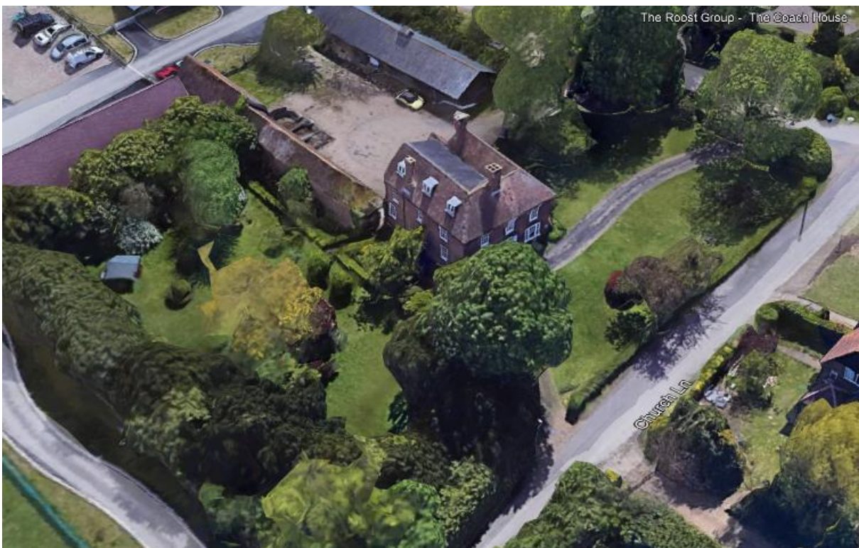
Site Visit Photo of Front Elevation:
