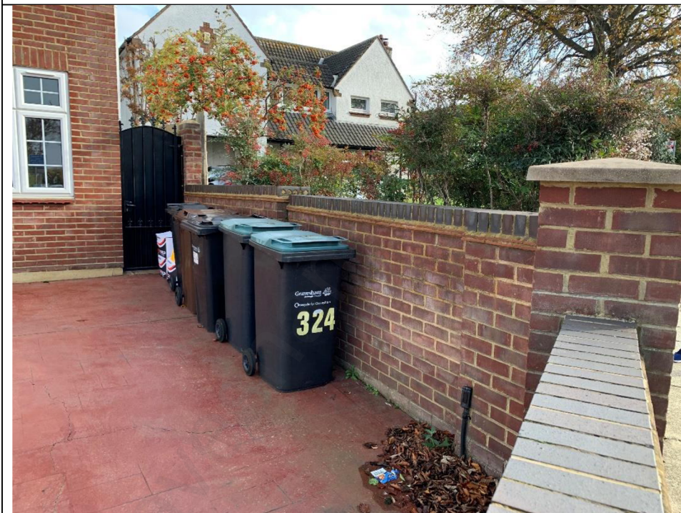
Lefthand side wall, east.
