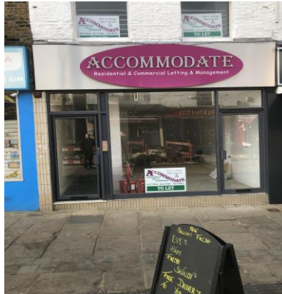
Site Visit (15 th February 2023)
