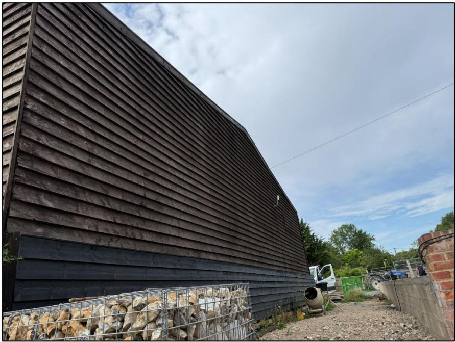
FIGURE 1-2 VIEWS TOWARDS THE EXISTING WESTERN ELEVATION OF THE BUILDING CONTAINING THE FARM SHOP
