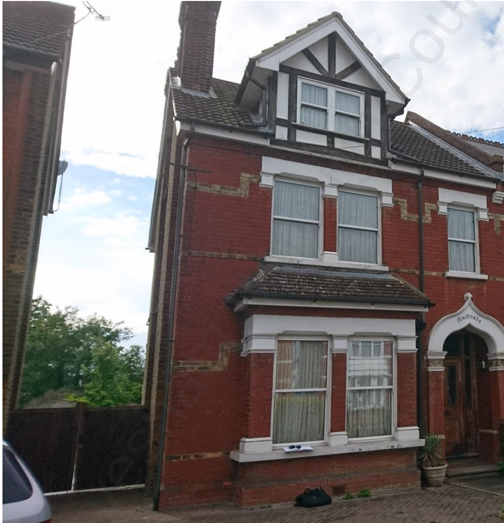
Front view of no. 124 Darnley Road, with shared rear side access to no. 126 to the left.
